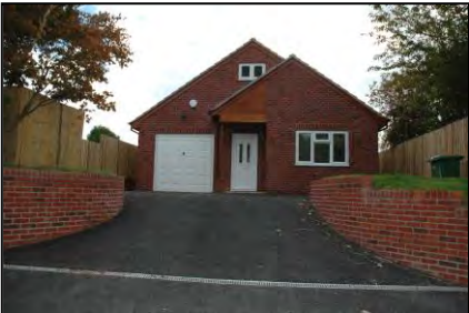
New build Bungalow Bishopstone
