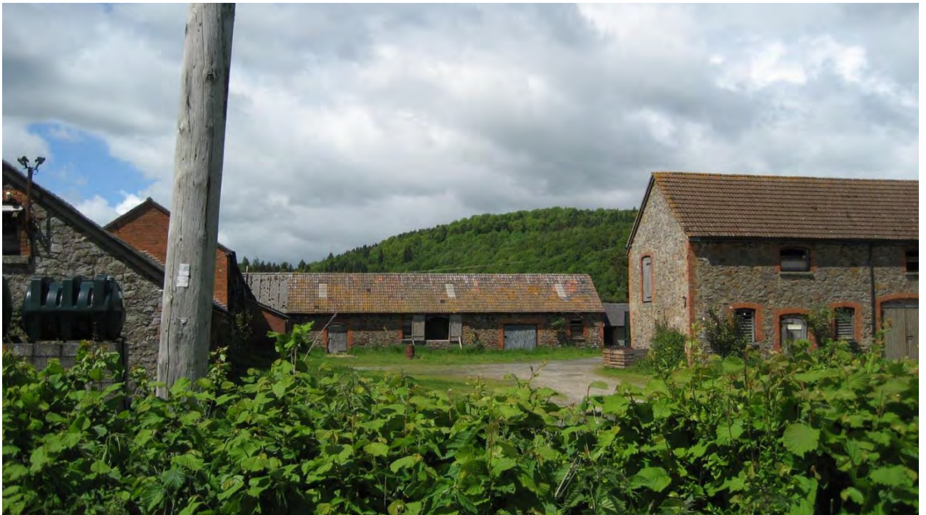
Figure 4 – Barn Complex at Brampton Bryan contributes to the Village's Character and Distinctiveness
