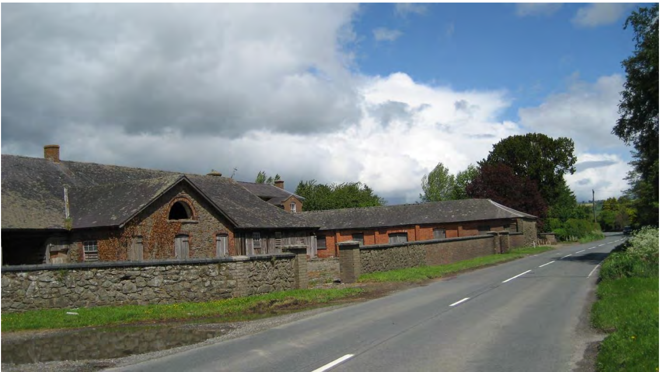
Figure 2 – Redundant Barns at Walford
