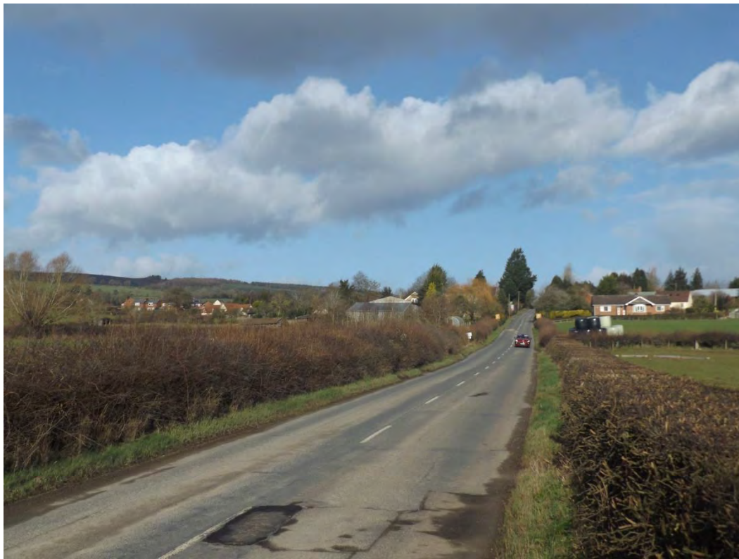
Figure 6: Approaching Richards Castle village from the south.
