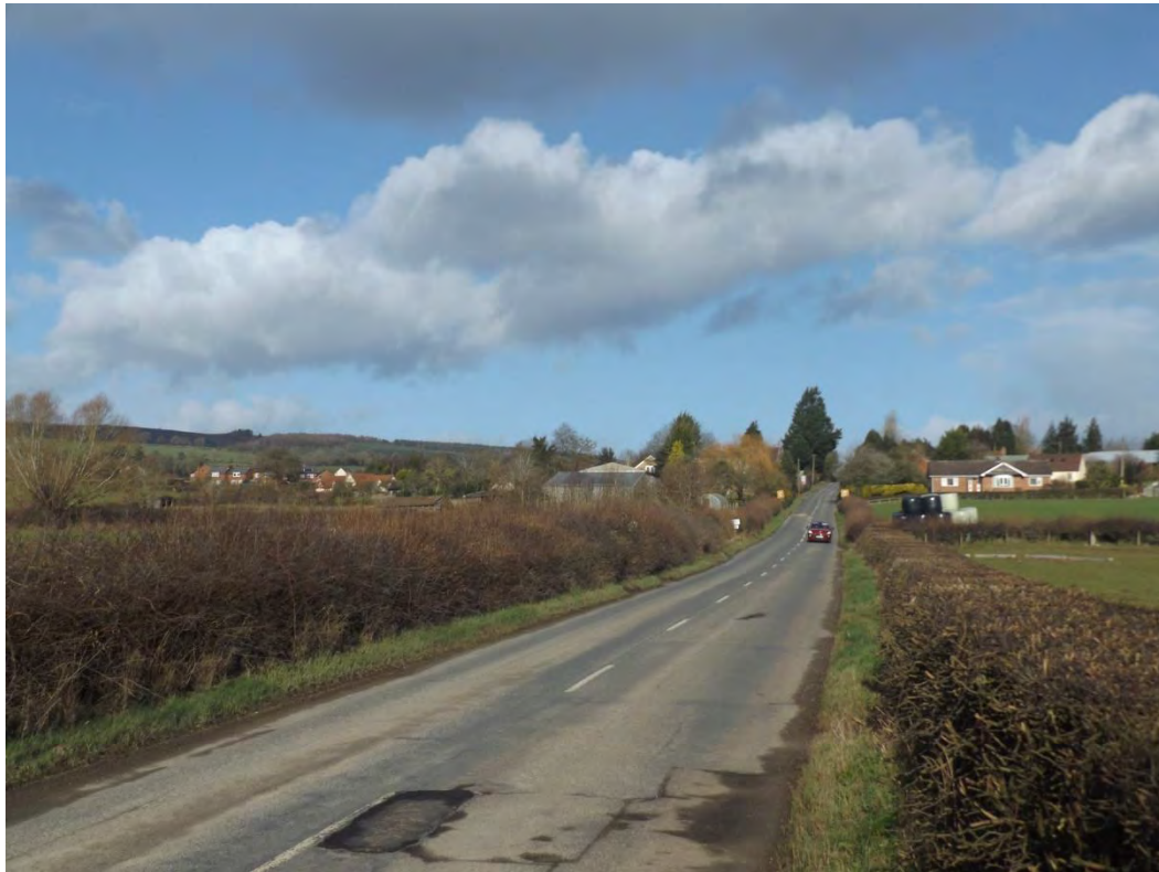
Figure 6: Approaching Richards Castle village from the south.
