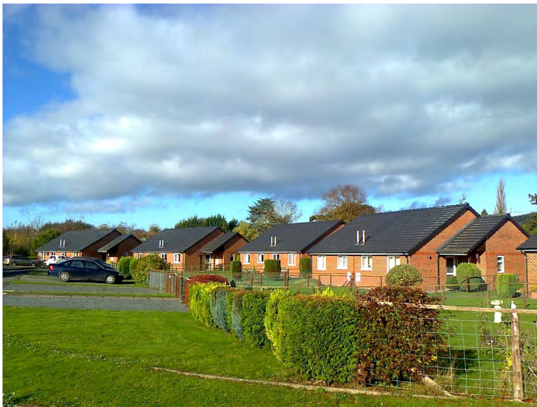
Affordable Housing Scheme, Barnfield
