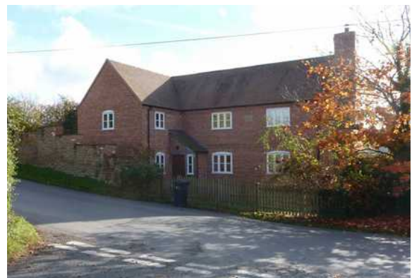
Nightingales – replacement of an old cottage Note the stone plinth and external chimney
