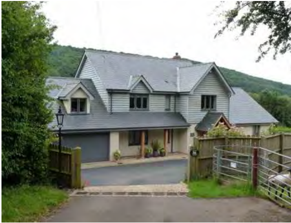
The main structure of this house is from the early 1970s; it was extended in 2000 and remodelled in 2009/10. The use of grey tiles and horizontal timber cladding in a lighter shade of grey together with other features gives a New England feel.
