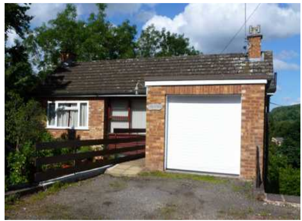
a split-level house making use of a steeply sloping site; gold coloured brickwork
