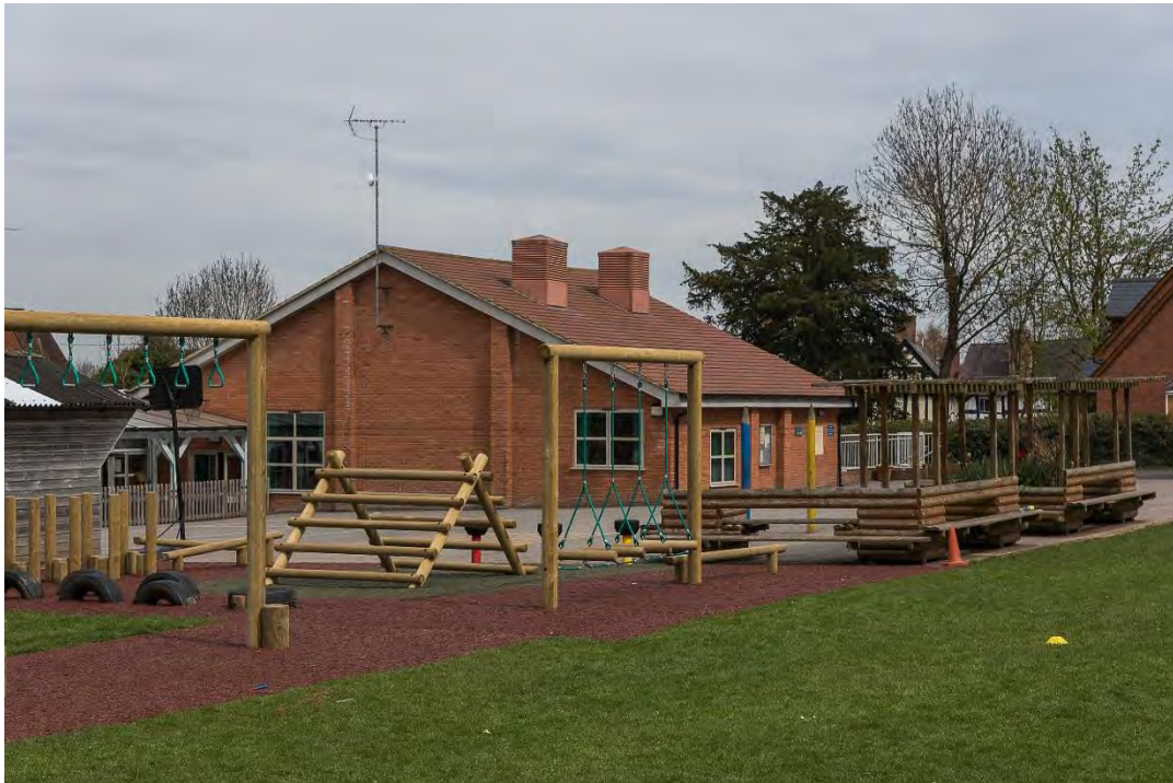
Figure 1 - Pembridge Primary School
