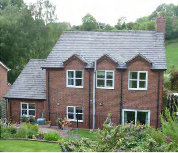
Built in 2001, the impression of dormer windows in the roof gives a cottagey feel.
