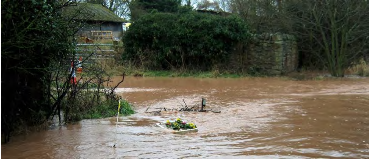
Flooding on Watery Lane
