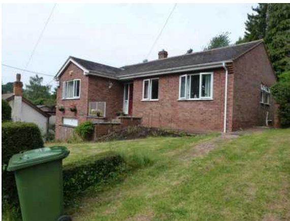
typical 1970s bungalow with basement garage similar to those at The Swallow
