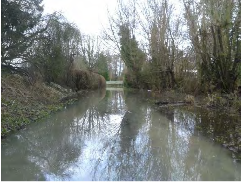
Figure 9 – Flooding is a major constraint at Walford (Looped Lane off Lingen Road - February 2014)
