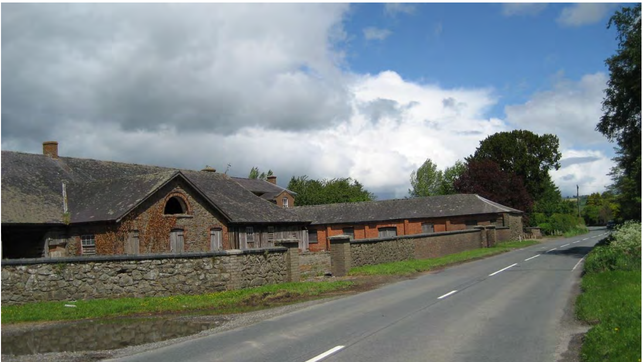
Figure 2 – Redundant Barns at Walford
