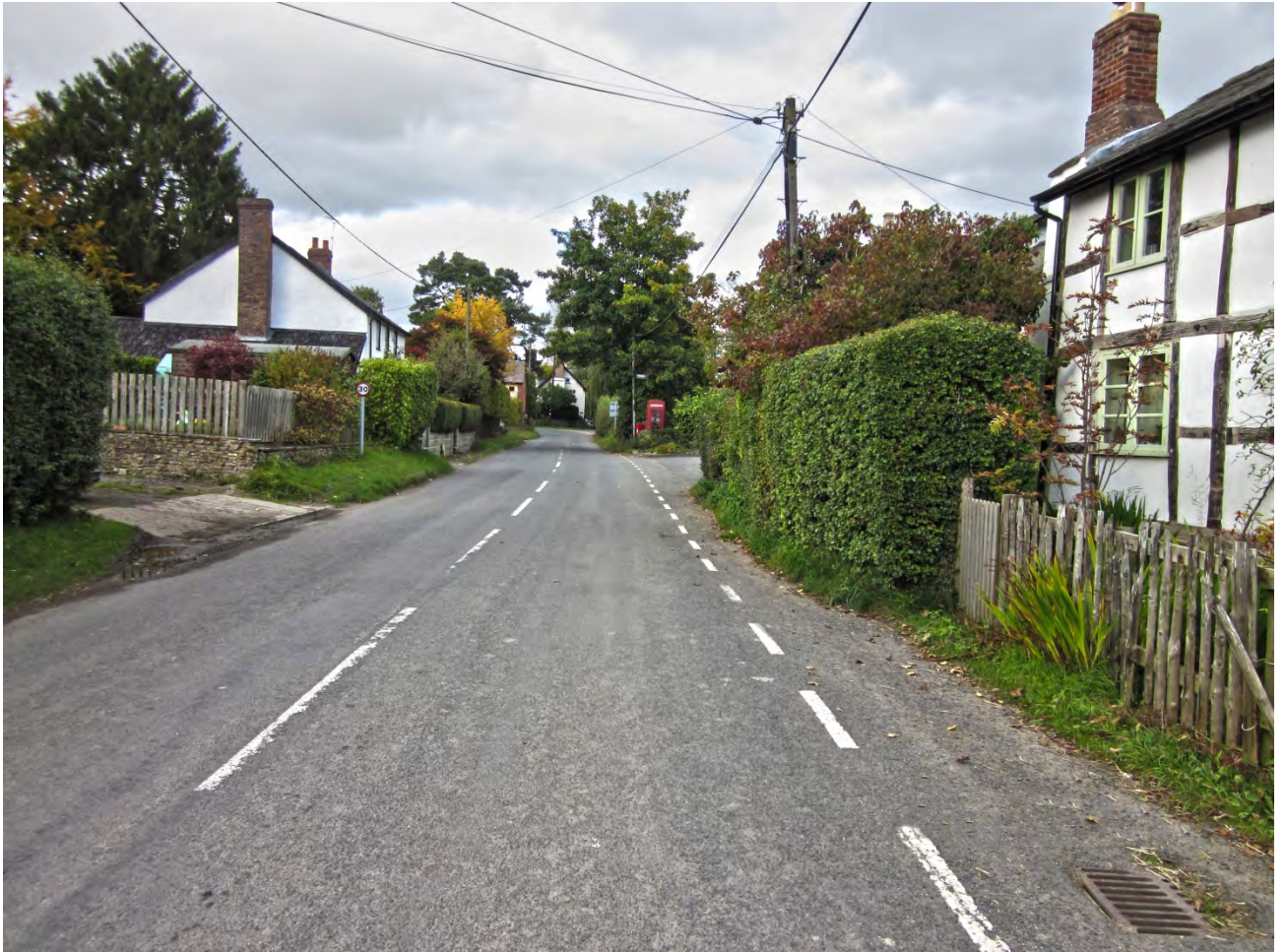
Figure 5 - Lingen looking north through village from the Bridge
