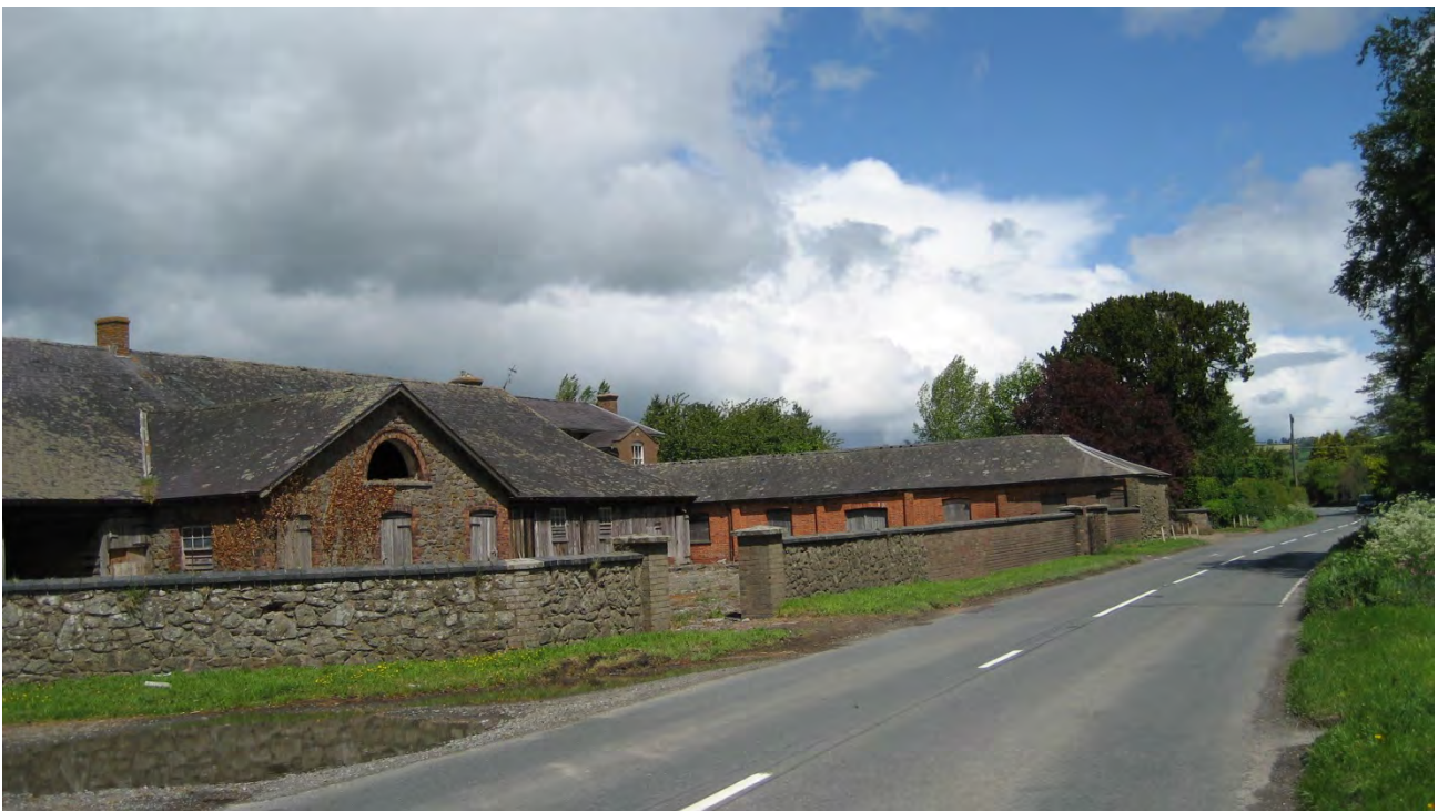
Figure 2 – Redundant Barns at Walford
