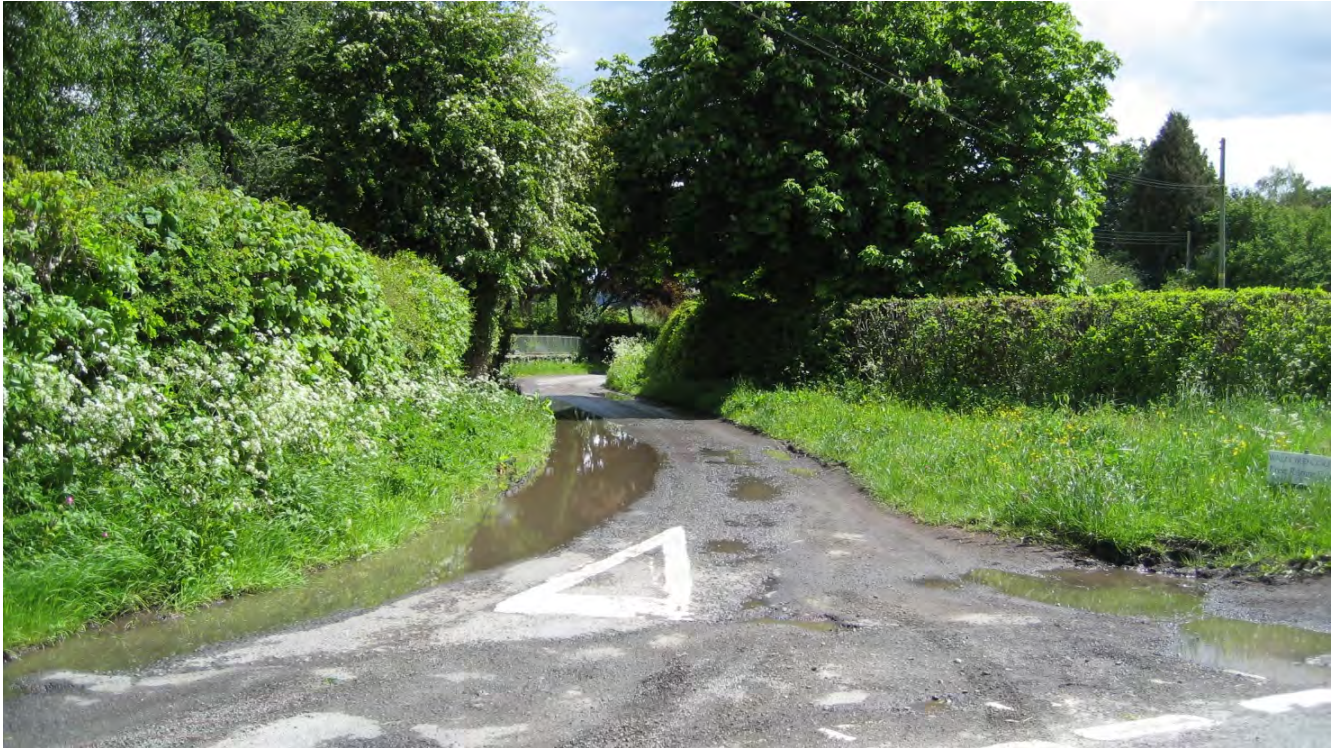
Figure 9 – Flooding is a major constraint at Walford
