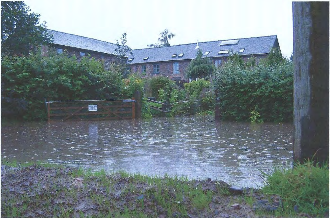
Photograph 2 - Flooding at Entrance to Fold Cottage
