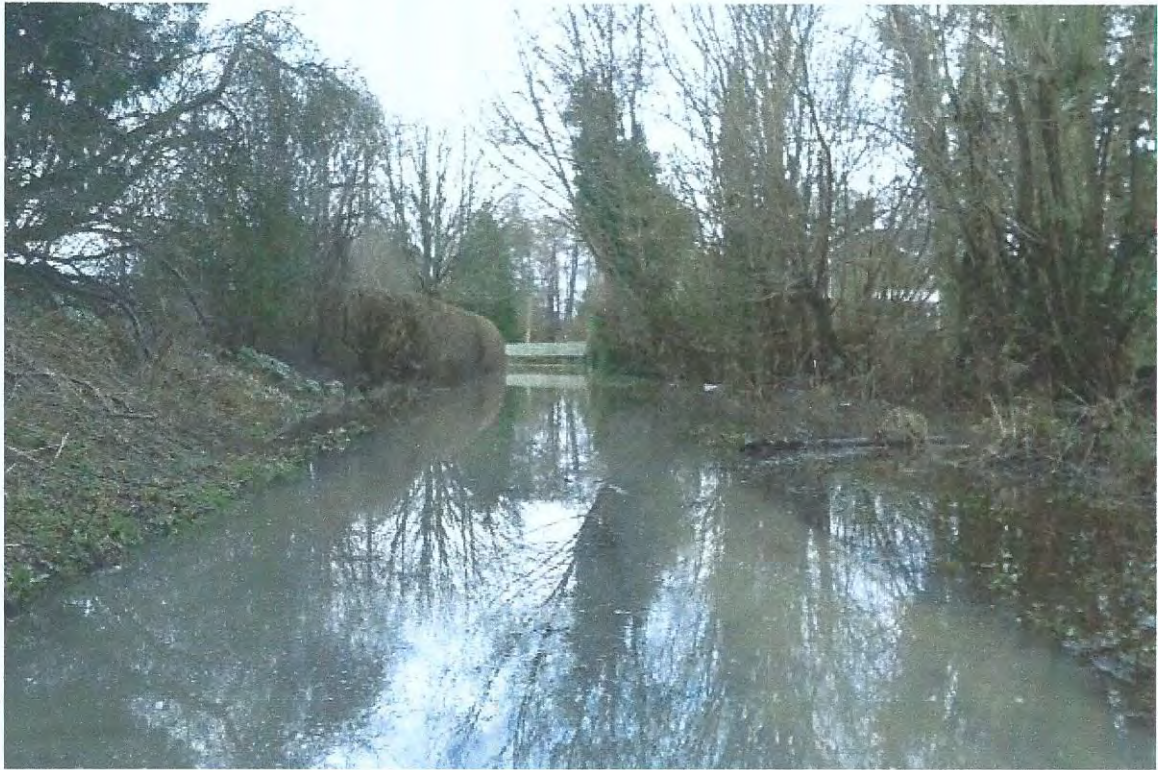
Photograph 1 - Flooding of Access Lane
