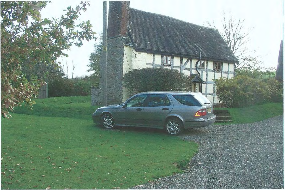
Photograph 7. Earth Bund to Around Fold Cottage
