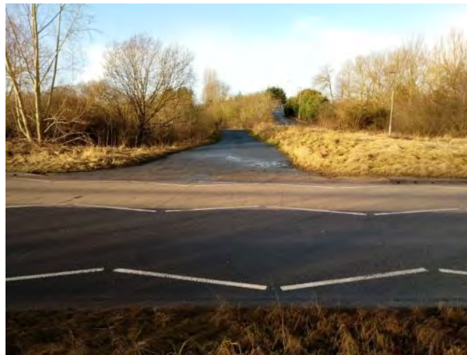
Existing Site Access
