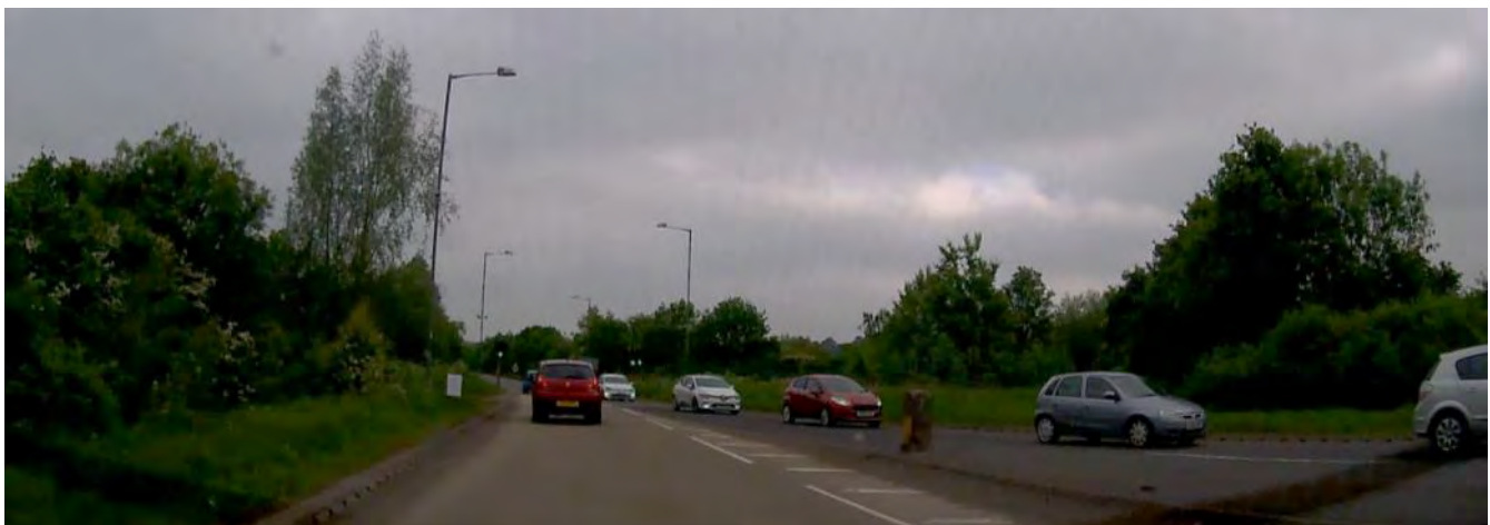
Visibility of the access (northbound direction)
