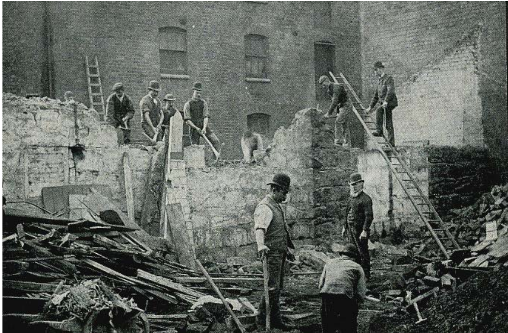
Alfred Watkins' photographs of the demolition of the city wall on the Old Wellington Inn site (now JDs) c.1900 immediately west of Widemarsh Street. The masonry was of 'primary build' type with large square blocks and small levelling-up courses. The photograph below shows a doorway found in the wall, probably late medieval
