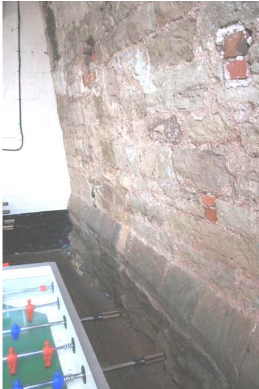
Detail of the wall in the Barrels, showing the extreme outward lean and the chamfered ashlar plinth with foundation courses below
