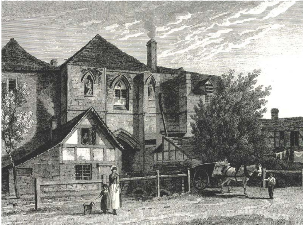
The exterior of the Bye Street (Commercial Road) Gate in the 1790s, from Duncumb's History & Antiquities of the County of Hereford
