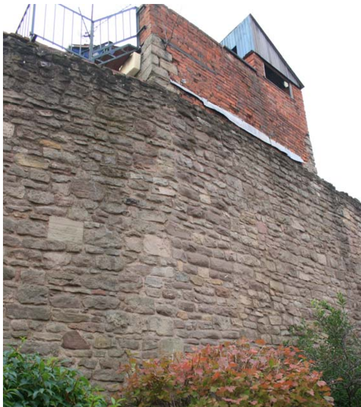
The Bastion Mews wall (exterior)
