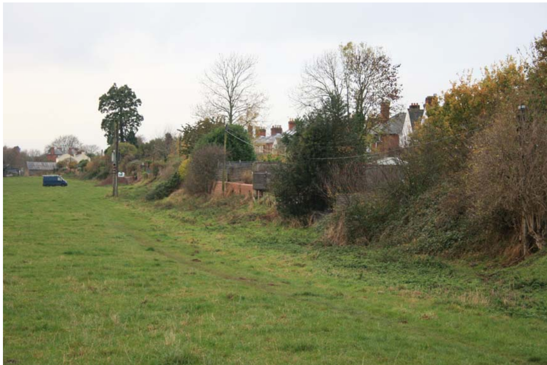
The Bartonsham Row Ditch, looking west from towards the east end of the monument
