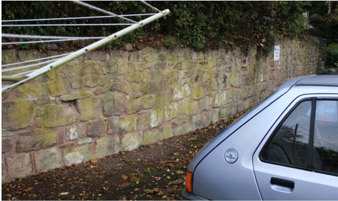
The wall, retaining the higher ground of the pre-Conquest ramparts, to the south of the Cantilupe Street excavation site
