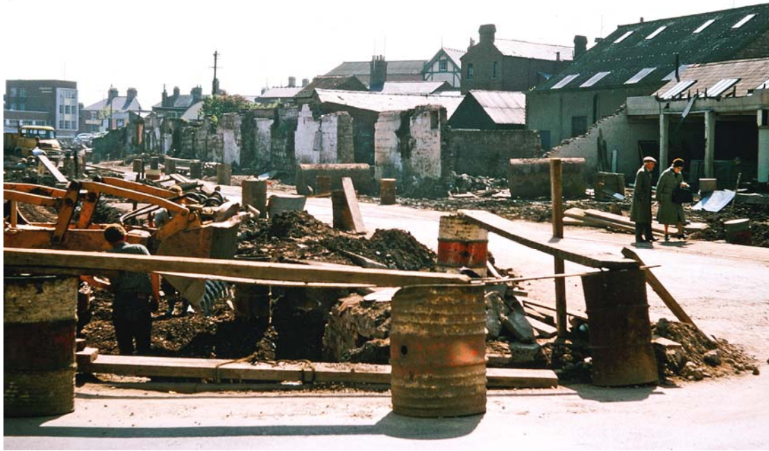
Blueschool Street in the 1960s, looking east, after the demolition of buildings on its south side revealed substantial sections of the city wall (Derek Foxtan)
