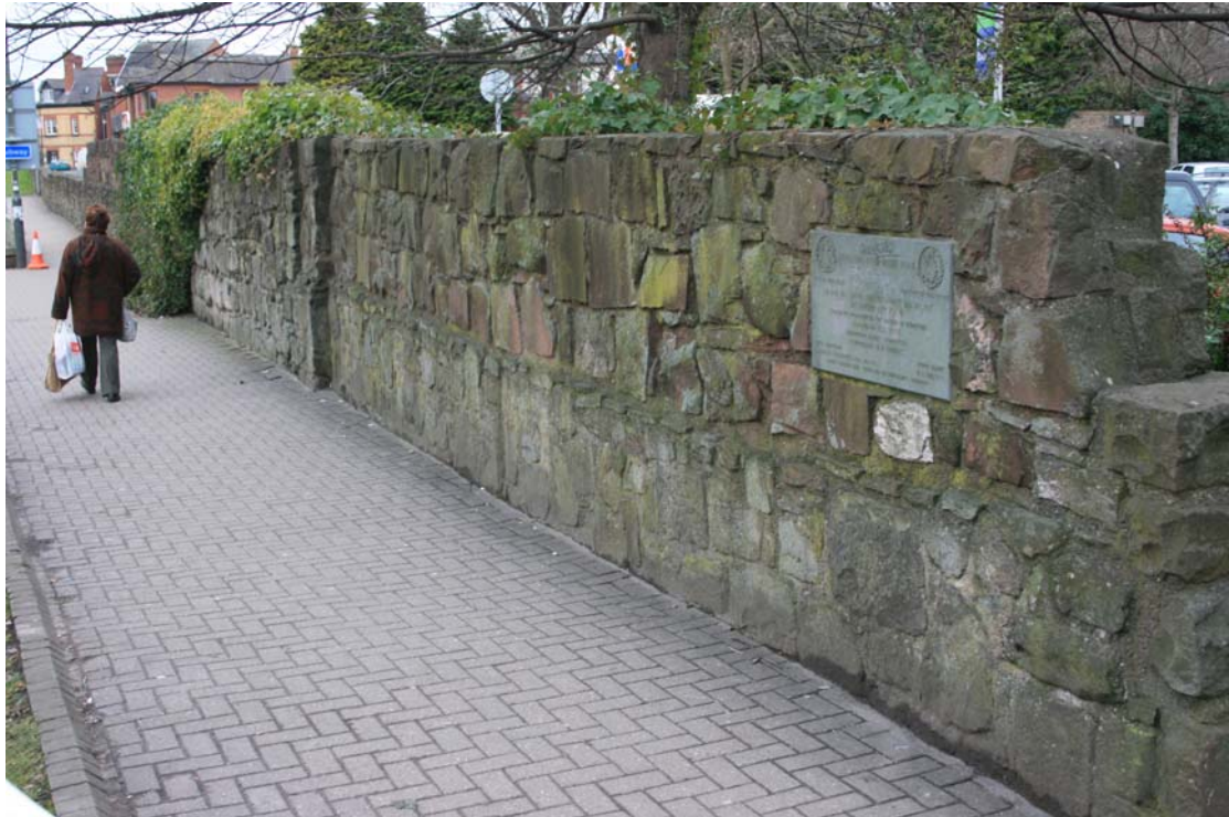
General view of the Wall Street section, looking east. The plaque in the foreground commemorates the opening of the Inner Relief Road in 1969 but is embedded in masonry of the c.1983 build. The lowest courses may be remains of the 1968 wall
