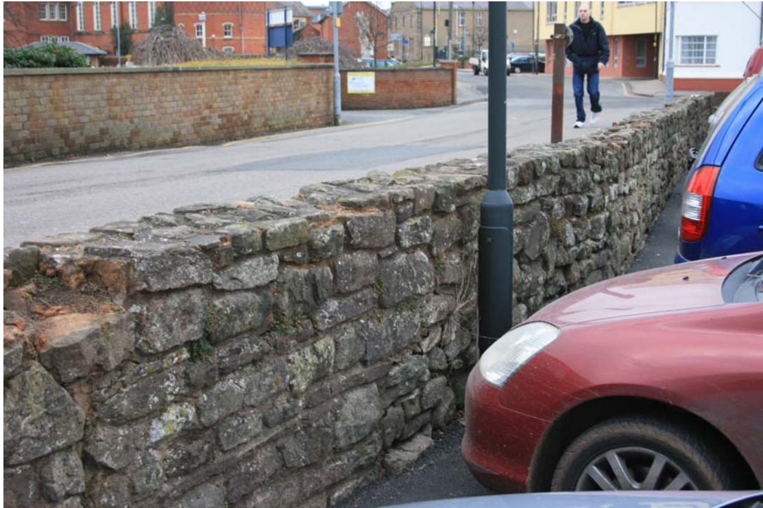
The Gaol Street/Bath Street car park wall, looking west (above), east (below). The wall beyond the lamp-post (above) is entirely modern; in front of the lamp-post the more regularly coursed masonry picks up the line of the medieval city wall. Gaol Street behind is at a higher (rampart-top) level than the car park (in the ditch)
