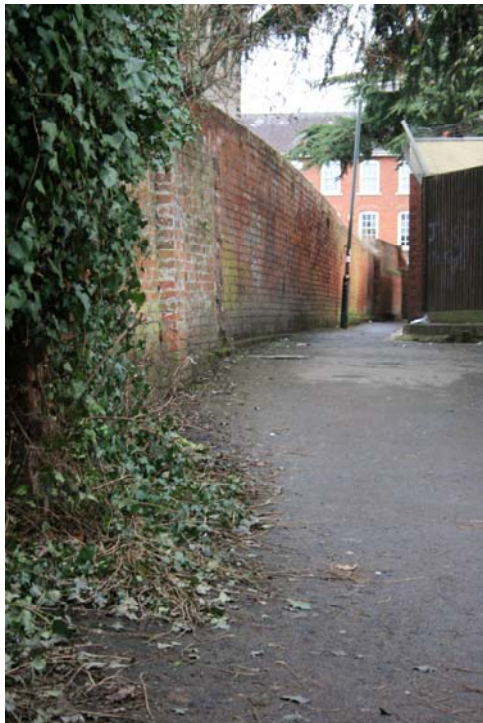
Levels dropping into the infilled ditch of the Bishop's Meadow Row Ditch to the north of Drybridge House at the rear of the St Martin's Street plots
