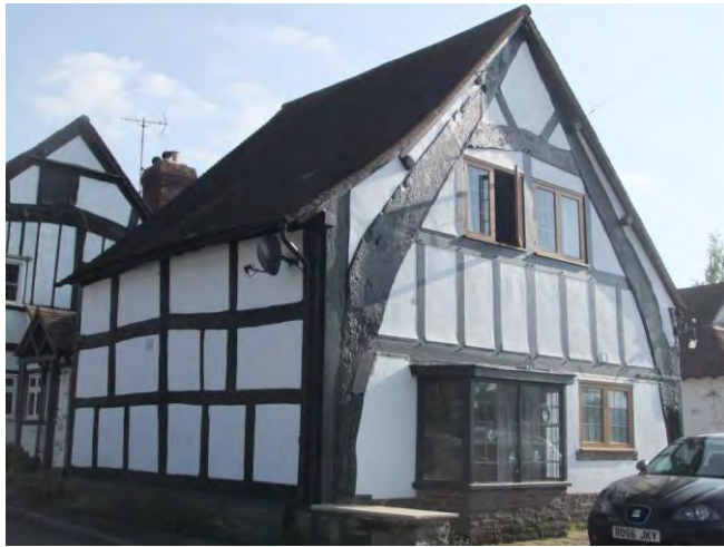
The Cottage, Church Road
