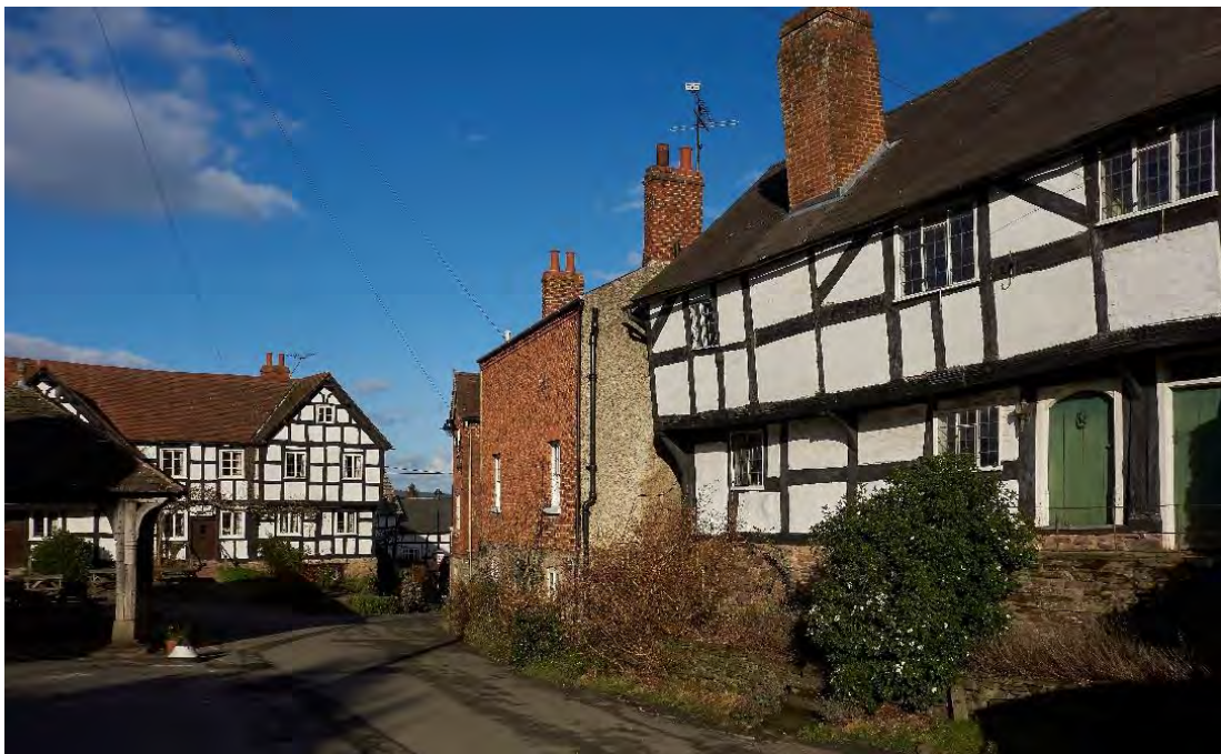
Figure 5 – Restricted road width within village core along Bearwood Lane.
