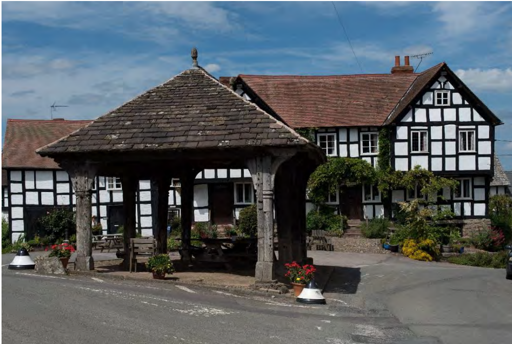
Figure 10 - Pembridge Market hall and The New Inn
