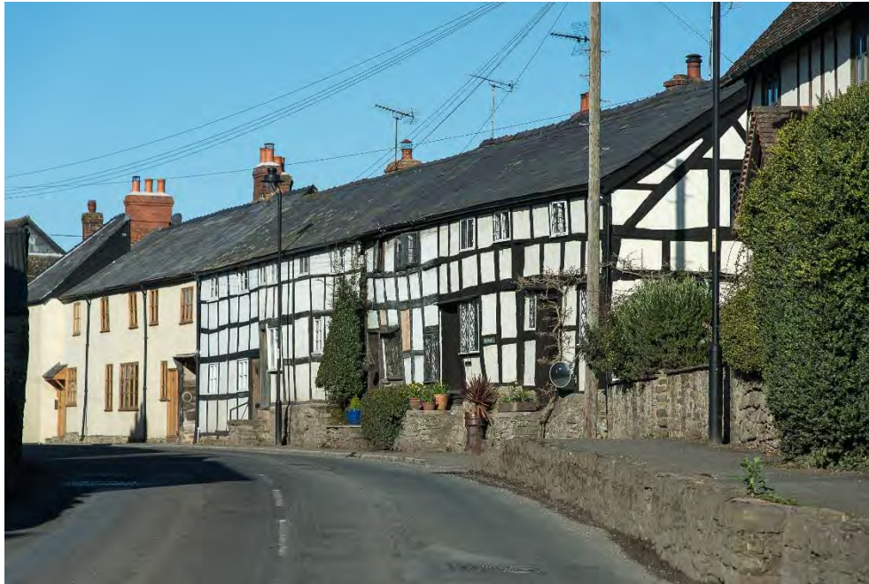
Figure 11 – East Street frontage
