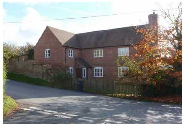
Nightingales – replacement of an old cottage Note the stone plinth and external chimney
