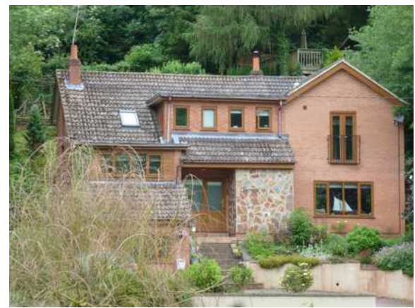
another house with tan coloured window frames; this time with a stone panelled porch; the 1990s saw some individuality of design, a movement away from the standardised 1970s and 1980s
