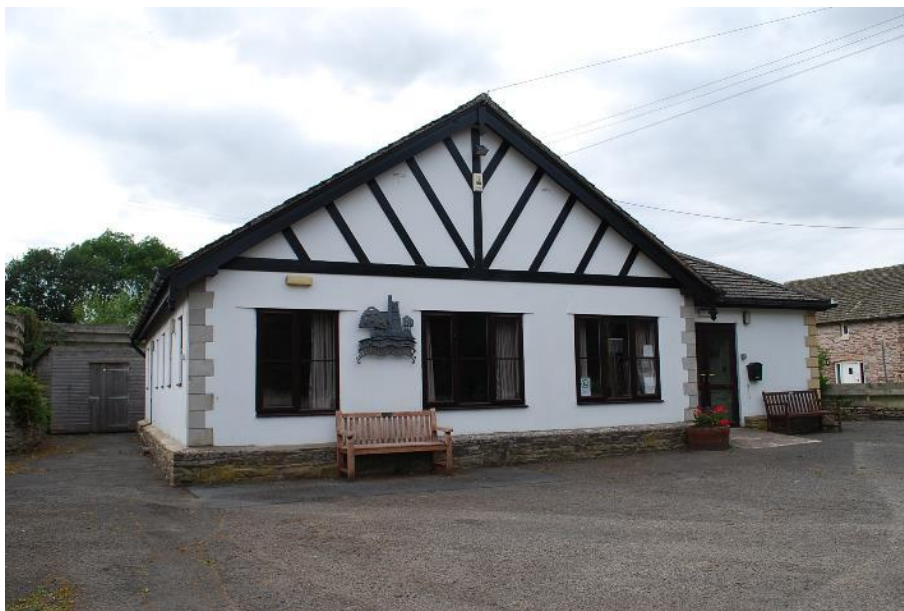
Figure 5 Staunton-on-Arrow village hall
