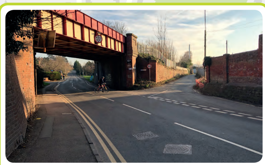
Existing railway bridge: To be signalled to allow space for footway/cycleway on northern side
