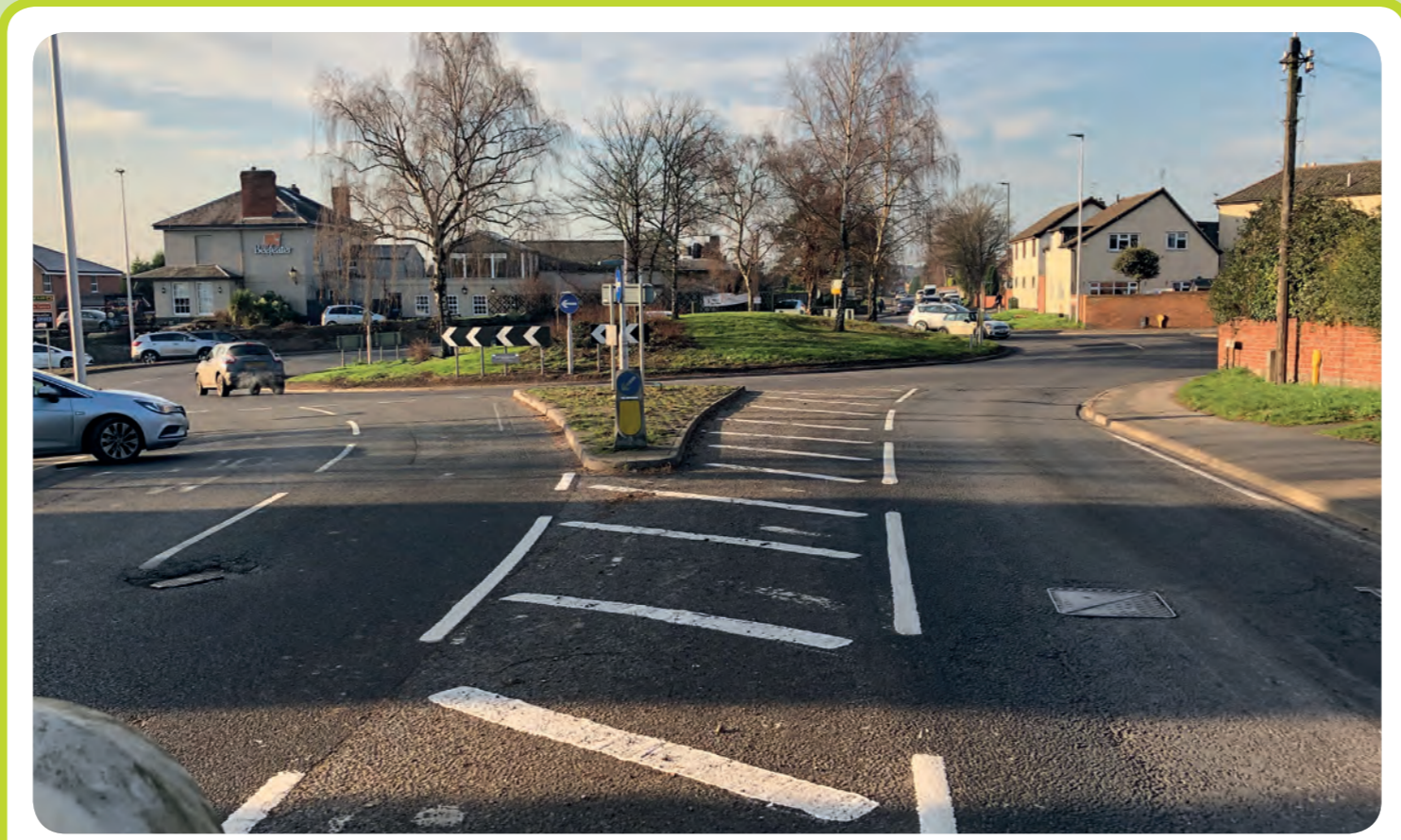
Safer crossings on all exits of Starting Gate Roundabout giving priority to pedestrians and cyclists
