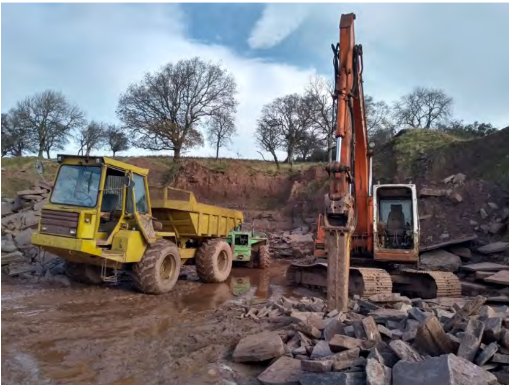
Photograph M17_2: Equipment within the site
