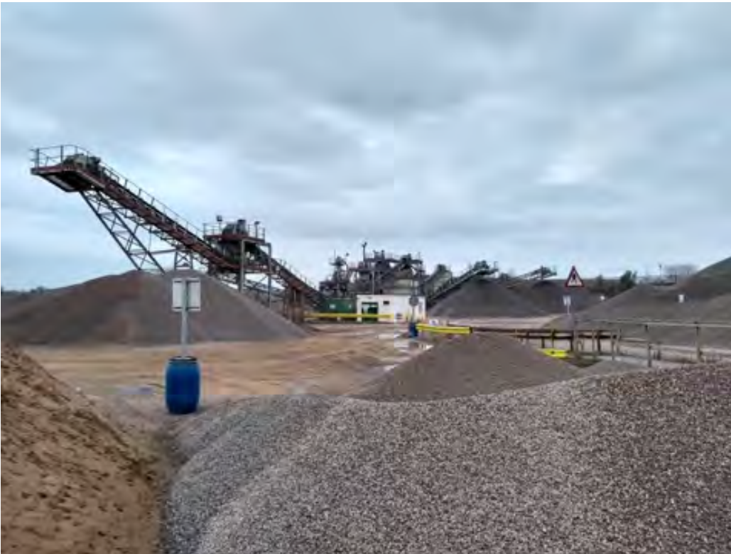
Photograph M05a_1: Minerals processing plant on site
