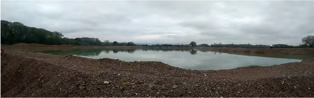
Photograph M05a_3: Working face
