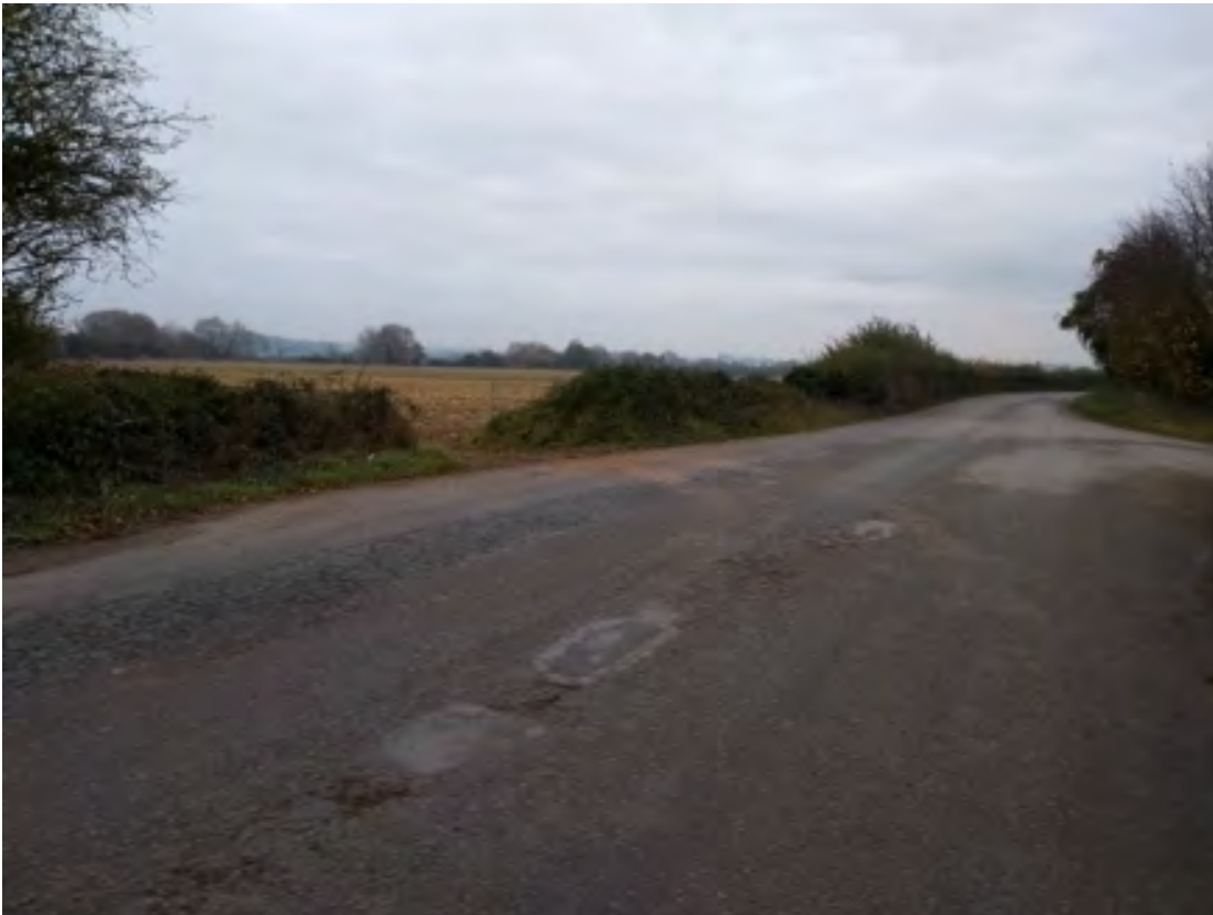
Photograph M05d_2: Road access
