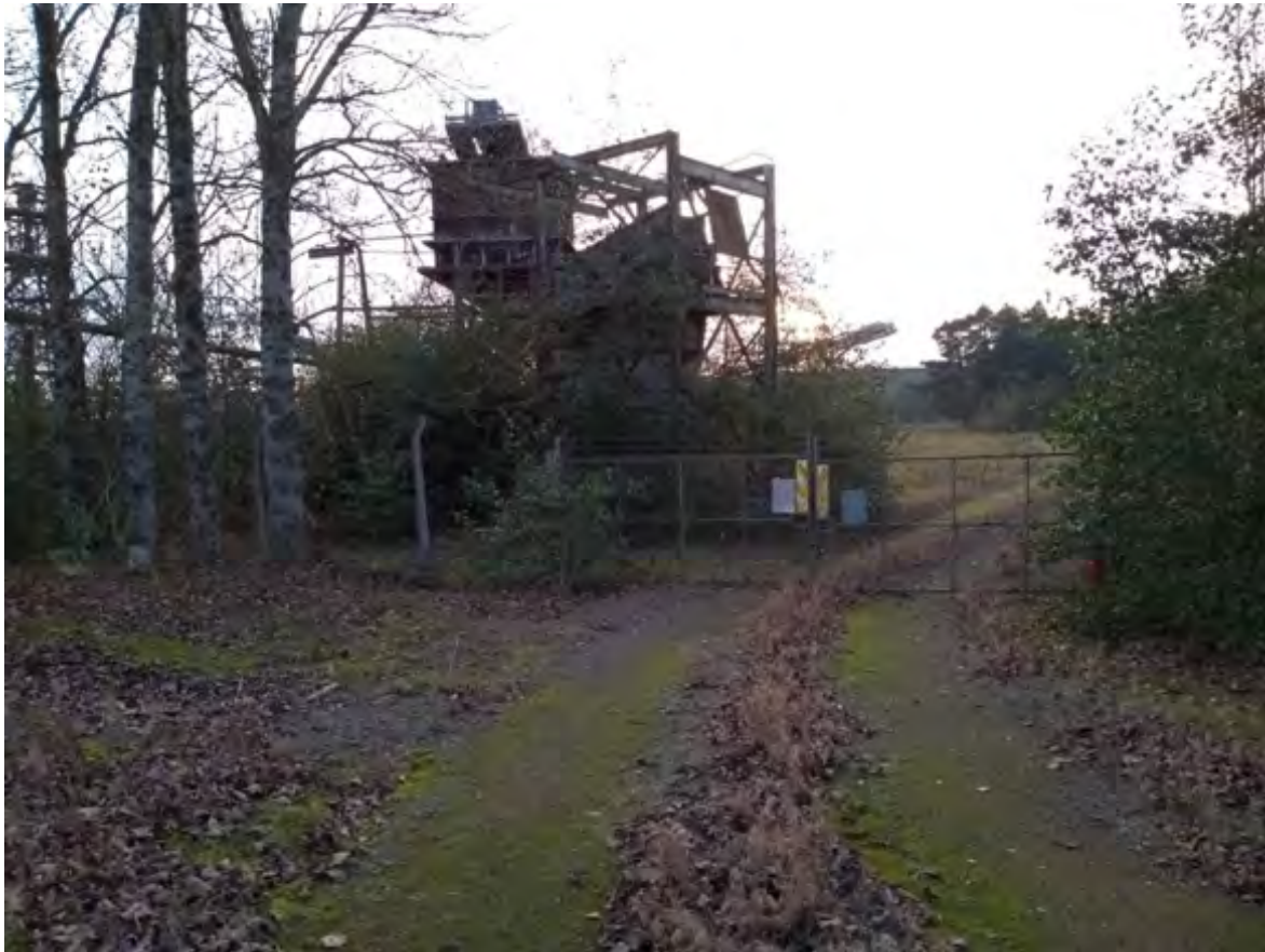
Photograph M04_1: Mineral processing plant on site
