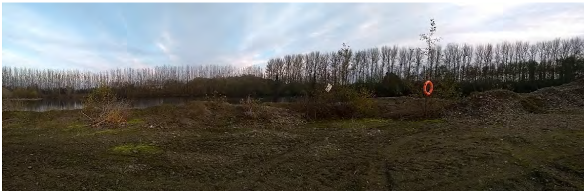
Photograph M04_2: Phase 1 restoration
