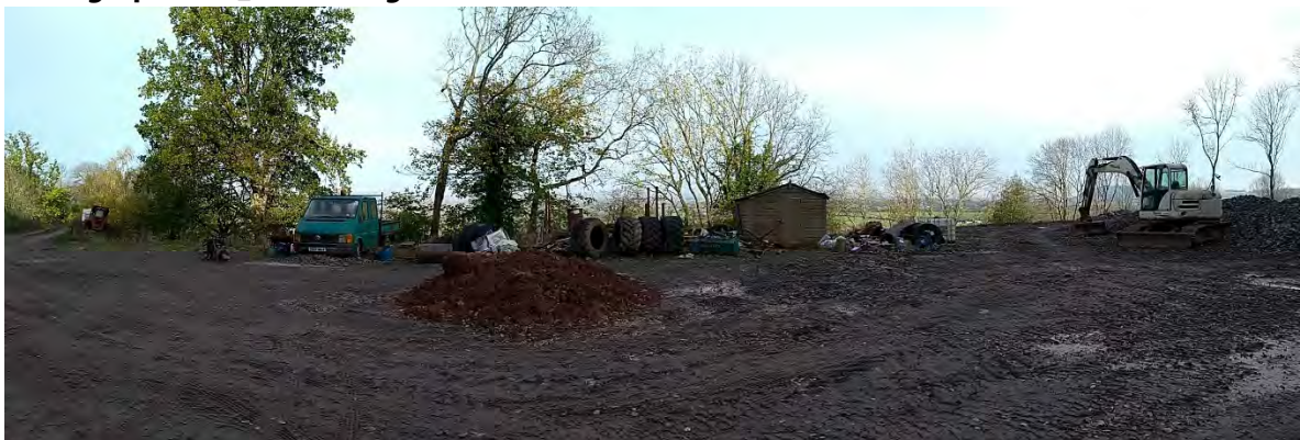
Photograph M20_4: Working area
