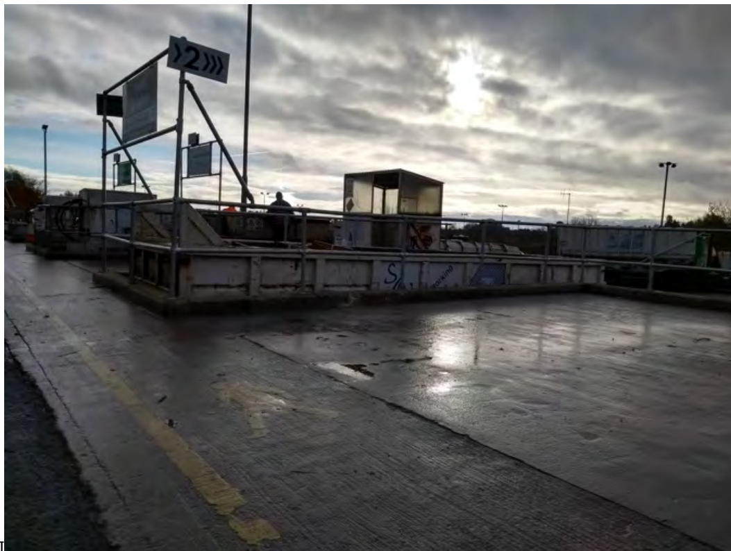
Photograph W05_2: View of site
