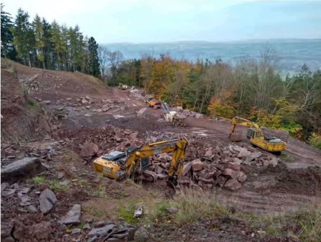
Photograph W57_1: Working face
