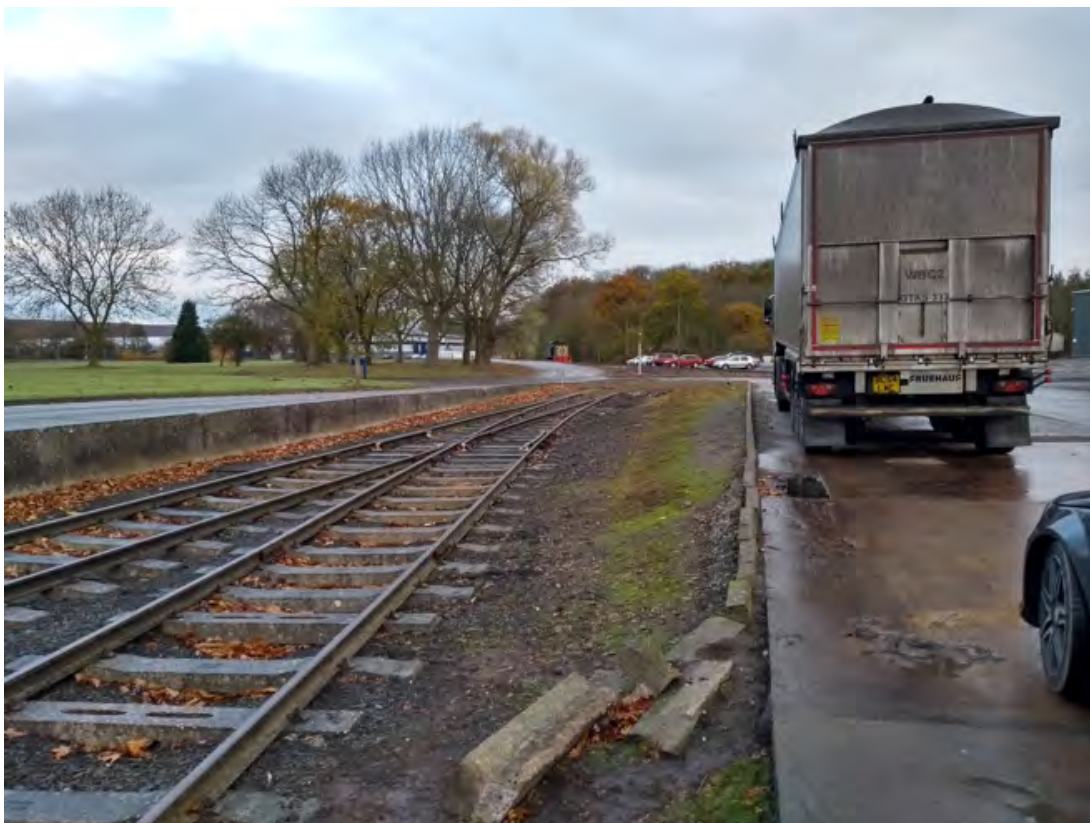
Photograph W66_2: Rail track into site
