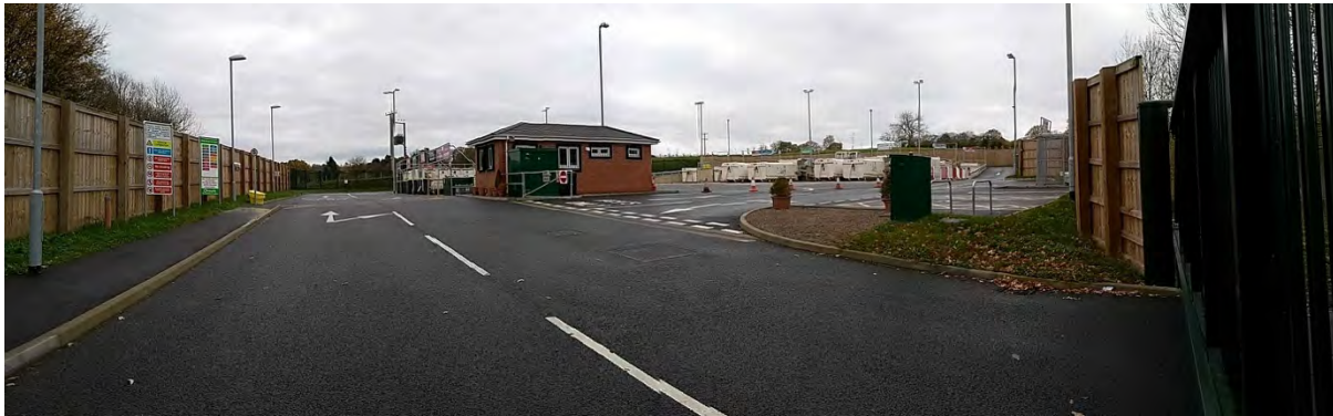
Photograph W10_1: View of site
