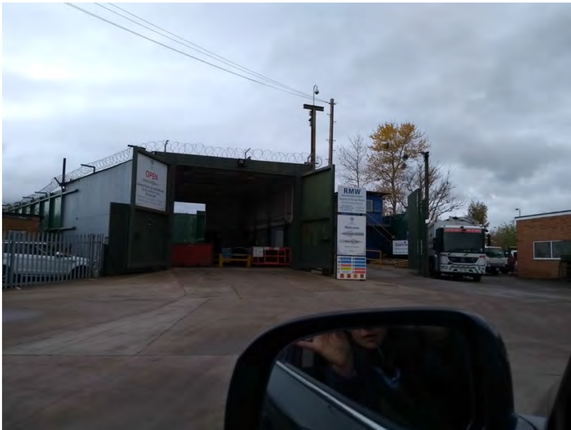
Photograph W22_1: Site entrance
