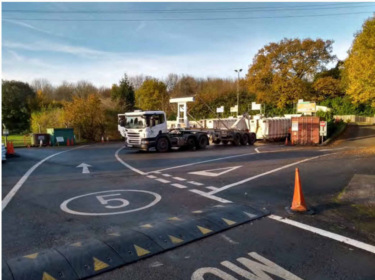
Photograph W07_1: View of site
