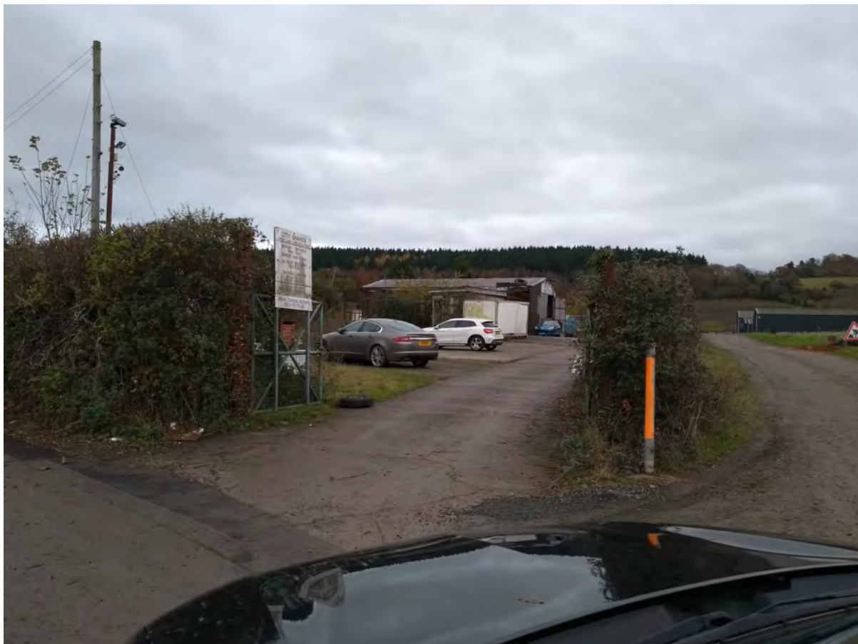
Photograph W19_1: Site entrance
