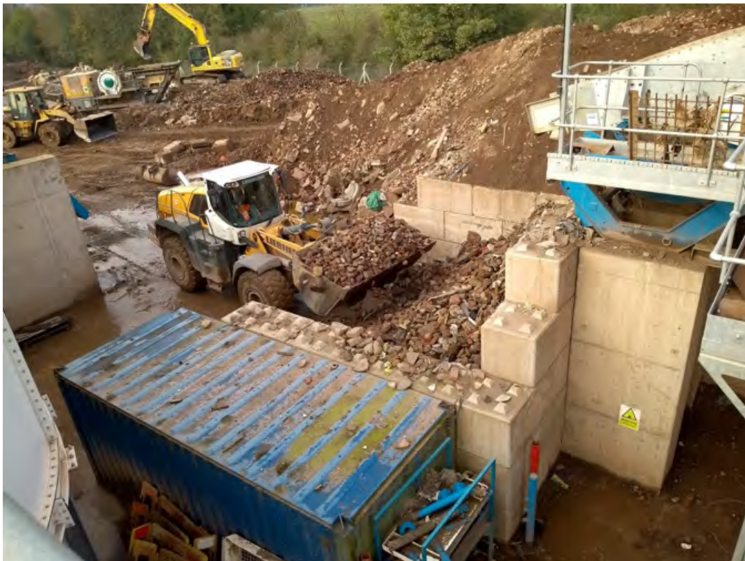
Photograph W13_2: Oversized material being taken off
