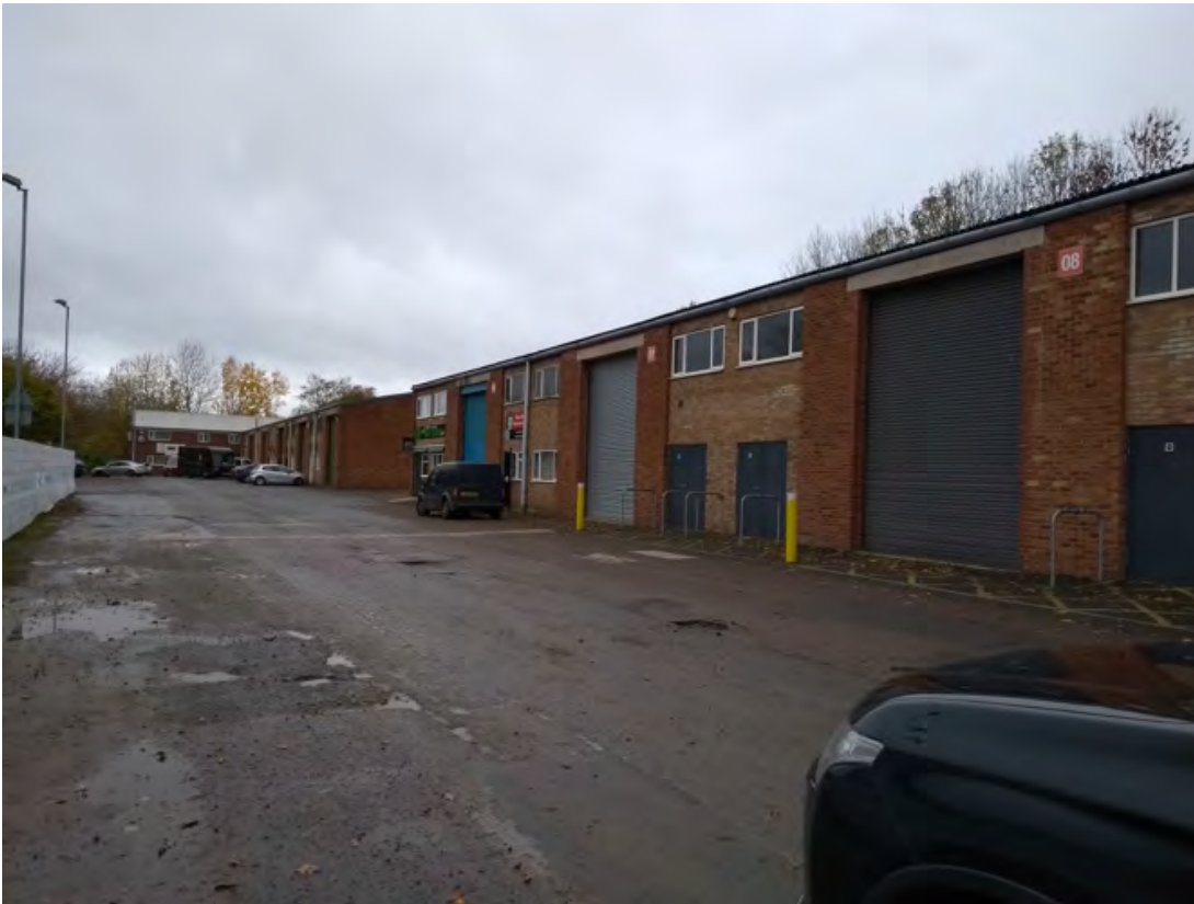
Photograph W60_1: View of site
