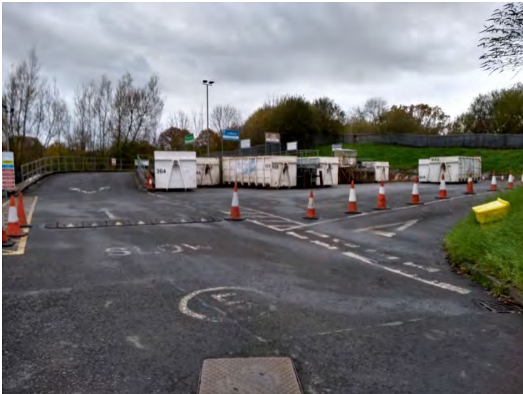
Photograph W09_1: View of site
