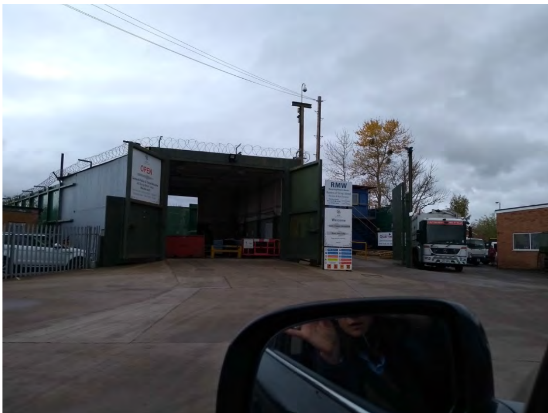
Photograph W23_1: Site entrance
