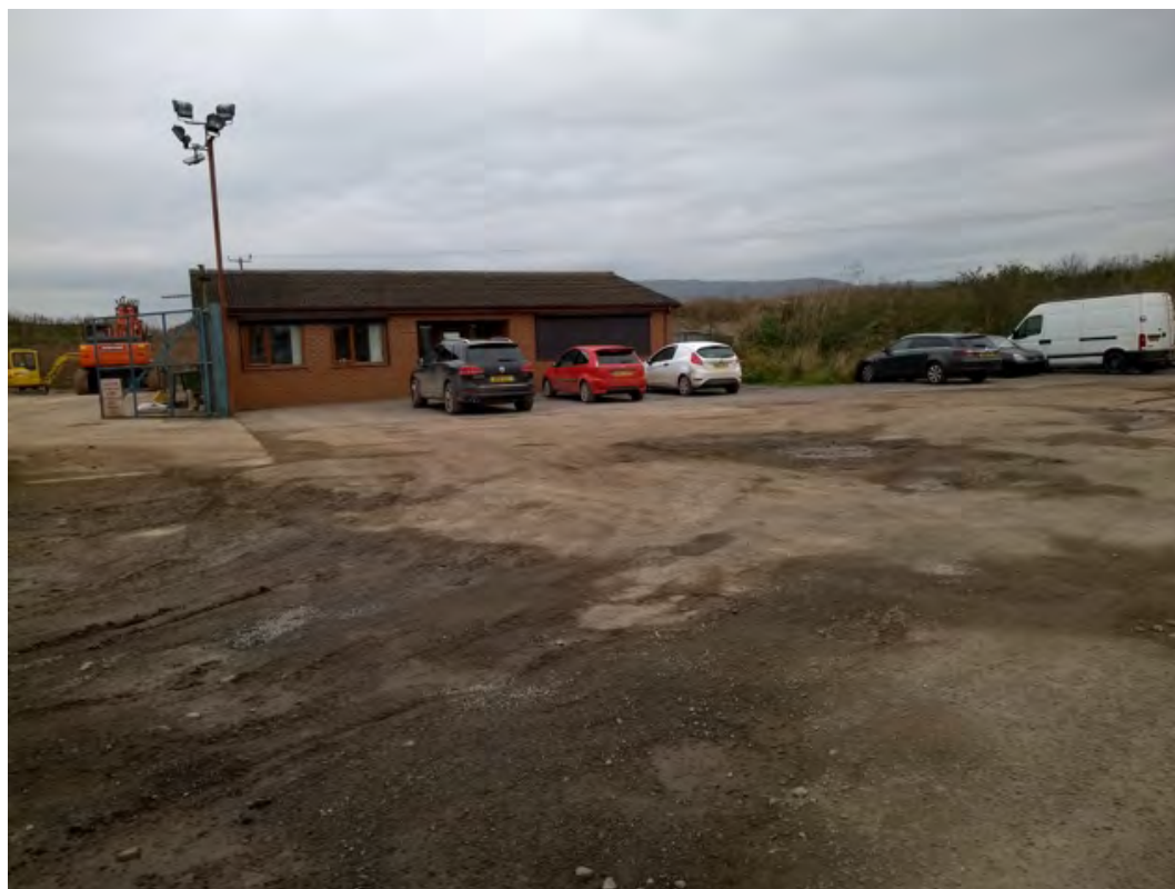
Photograph W11_1: New office on site, bunding to the right with materials processed behind.
