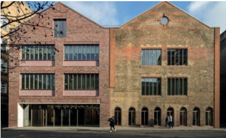
Contemporary interpretation of Victorian warehouse, Great Suffolk Street, by Hawkins Brown
