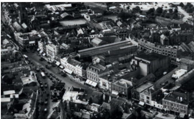
High Town c1950, detailed rooflines conceal larger massing behind
