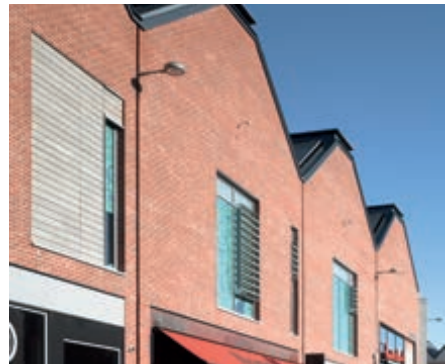
Roof articulation within Old Market
