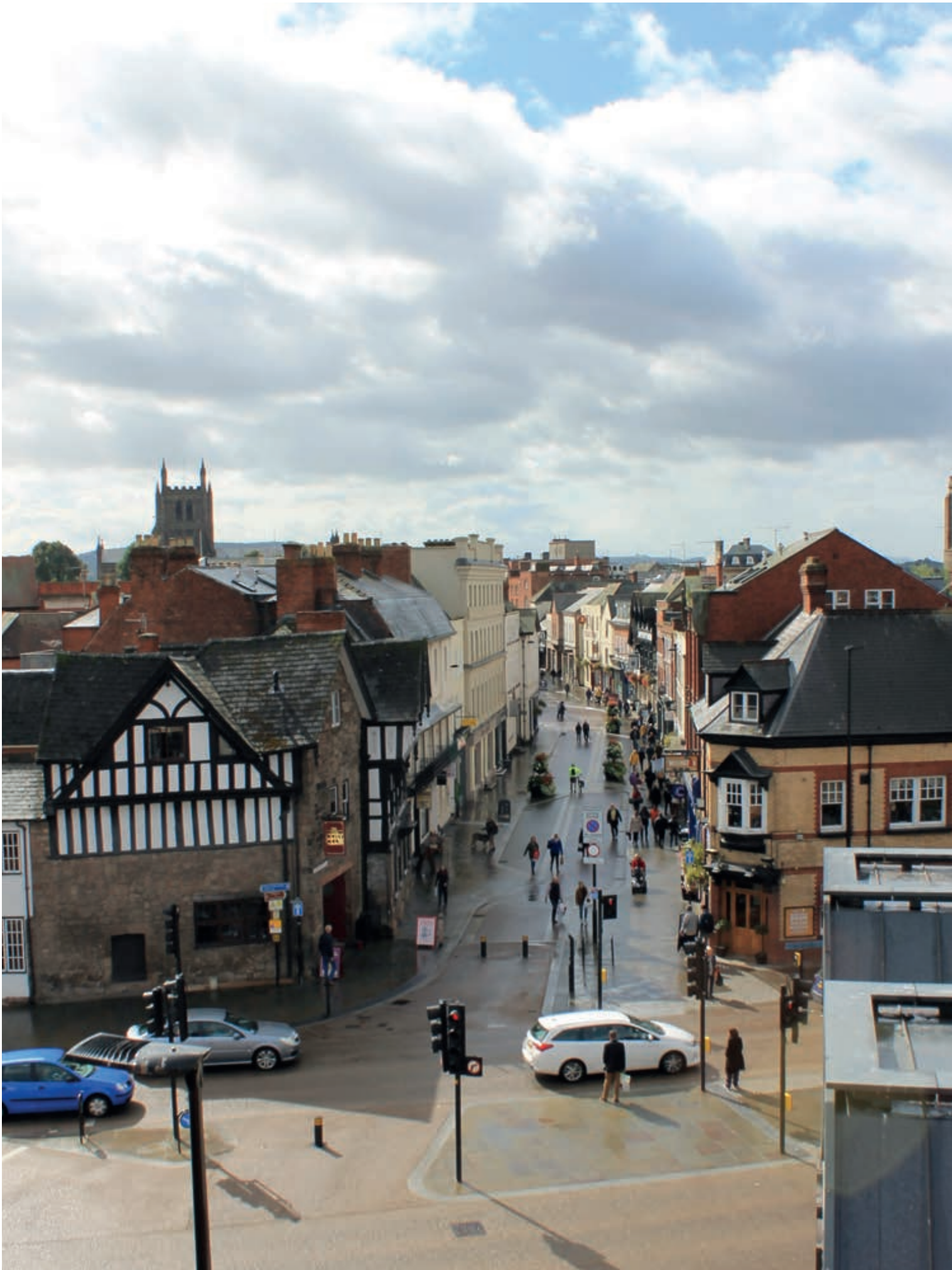
View looking south along Widemarsh Street from the roof of Garrick House Car Park
