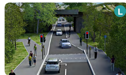
Signalised one way working over/under railway bridge
