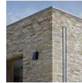
Recessed downpipes
