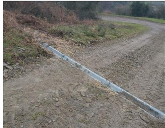
Figure 9-14 Cross drain – NFM Construction grant recipient (2021)
