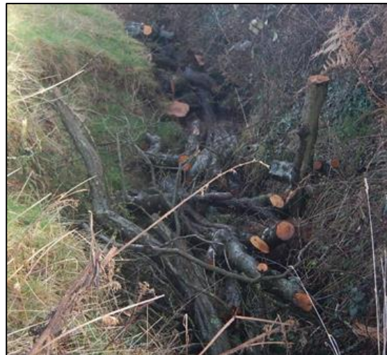
Figure 9-11 Natural in-ditch seepage barrier – Herefordshire Council (2020)
