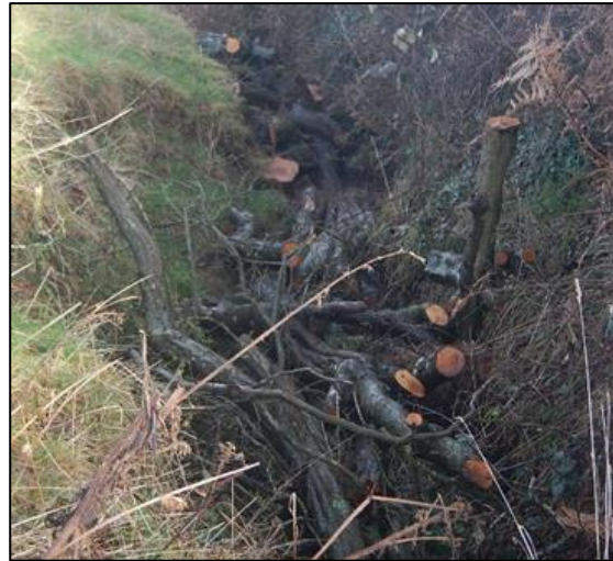
Figure 9-11 Natural in-ditch seepage barrier – Herefordshire Council (2020)
