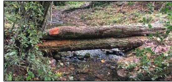
Figure 9-12 Leaky dam – River Wye and Lugg NFM pilot project participant (2019)
