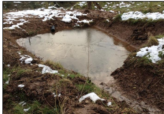
Figure 9-7 Sediment trap – Yorkshire Dales Rivers Trust - Tees Rivers Trust
