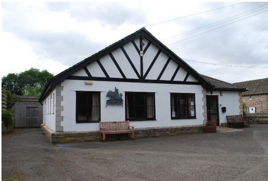
Figure 5 Staunton-on-Arrow village hall
