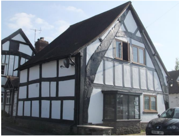
The Cottage, Church Road
