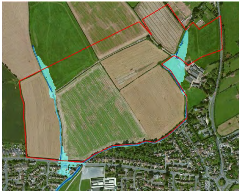
Fig 5.1. Holmer West Aerial Image (Taken From Bloor Homes Public Consultation Boards for Holmer West).
