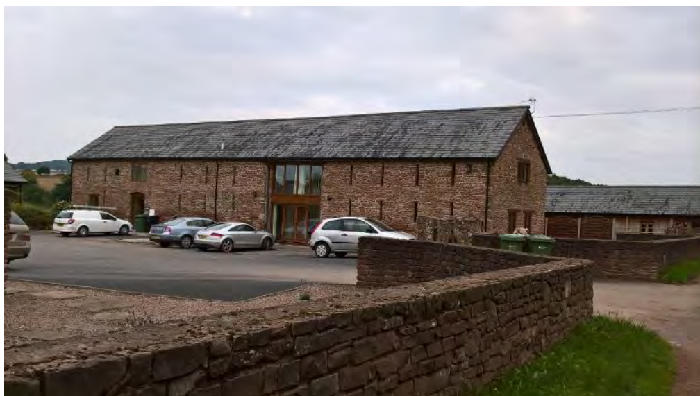
Converted rural building
