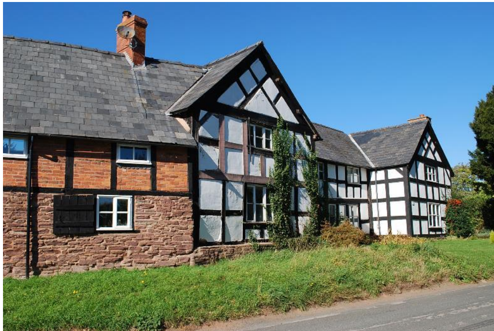
Grade II listed Church Farmhouse, Madley
