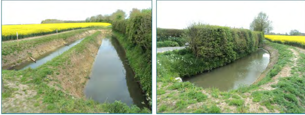
Figure 1: Images of U shaped and linear shaped silt traps installed in the Wensum catchment by Norfolk Rivers Trust and Norfolk Internal Drainage Board.
