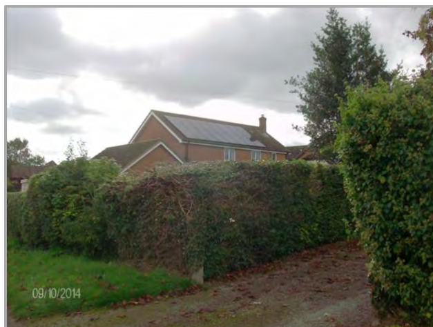
Solar Panels on a residential property in Llangrove
