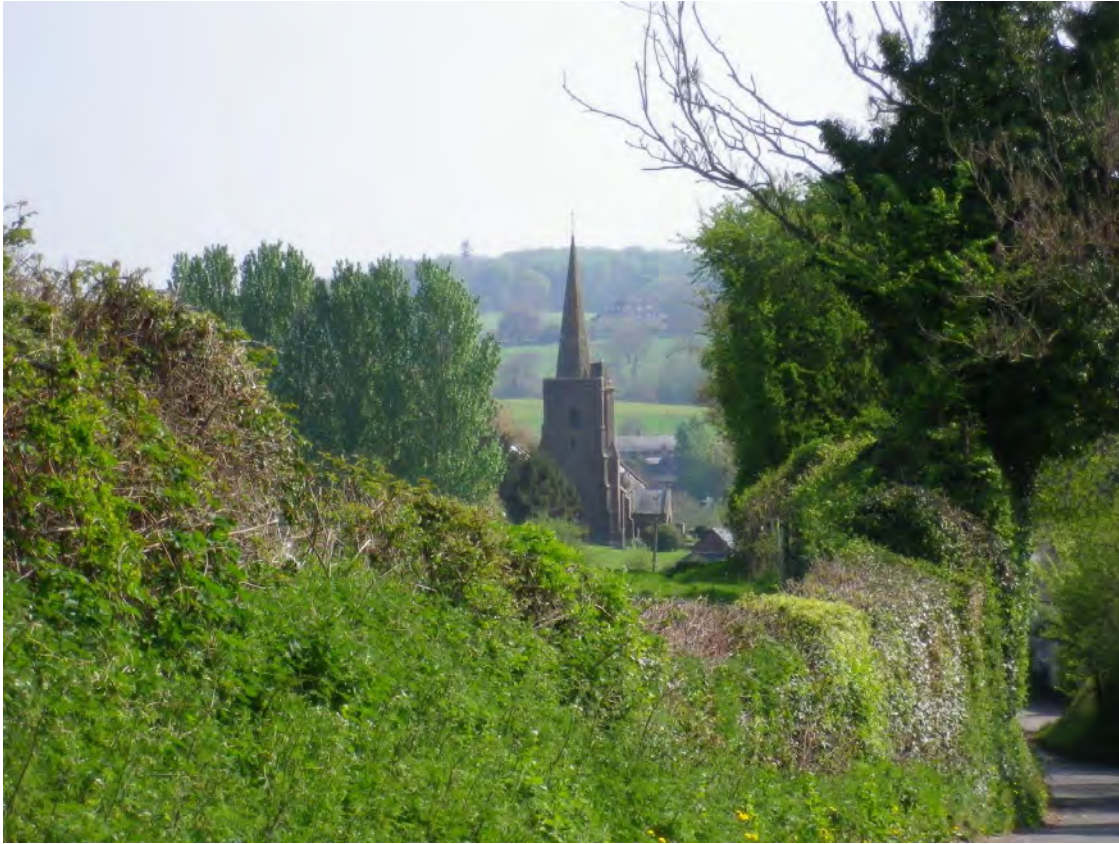
View 4: View of the Church approaching the village on the Llangrove Road (Number 4 on Map 3)
