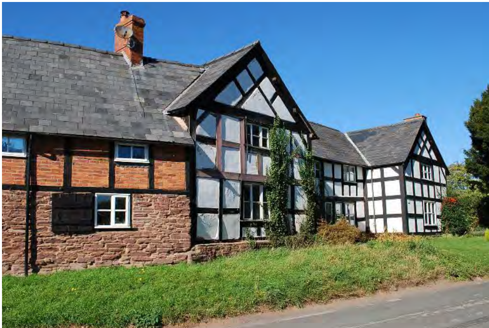
Grade II listed Church Farmhouse, Madley
