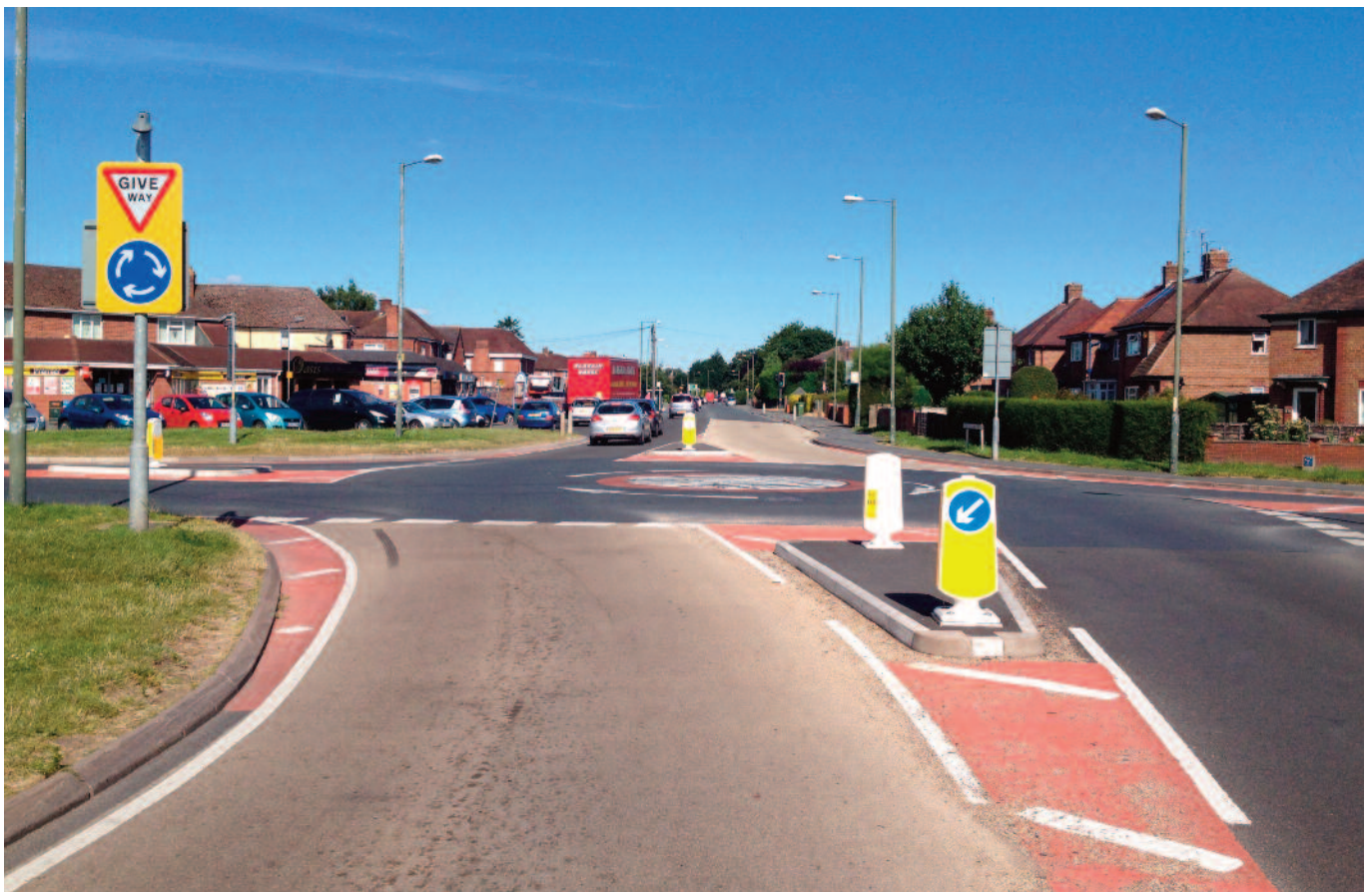
A recent road safety scheme on Holme Lacy Road.
