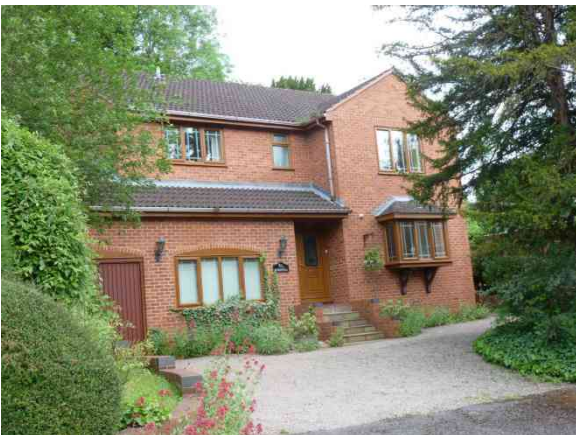
medium red brick and grey tiled roof with oriel window; house built in the 1990s; tan coloured window frames are a departure from the standard white; front window and garage have arched heads
