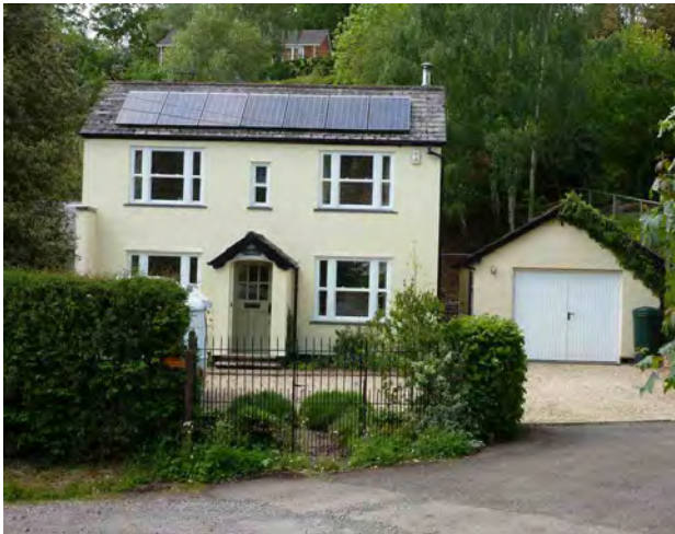
Greenbank - modernised to high standard Including exterior insulation
