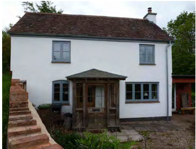
White Cottage - modernised to a high standard Including exterior insulation
