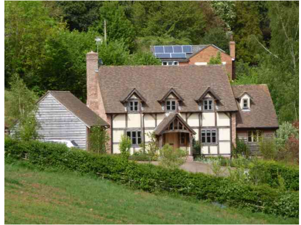
A Border Oak, timber-framed house built in 2007 in the valley off Pub Lane. A slightly different Mock Tudor design to the other development, the dormer windows give it a more cottagey look - similar in design to Windmill Cottage on Church Lane (see 'gabled dormer' on page 82).
