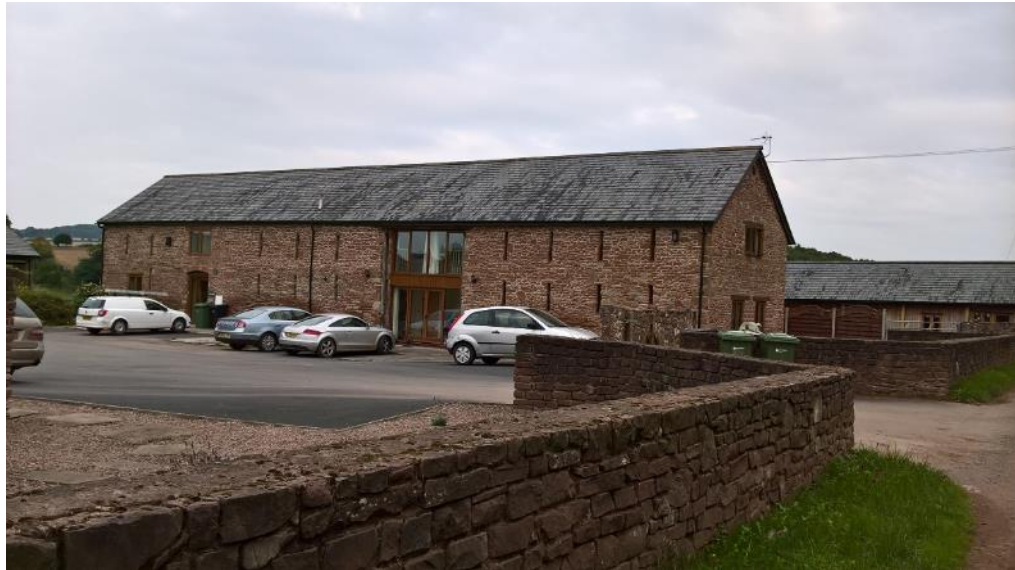
Converted rural building
