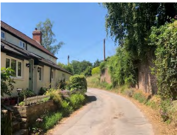
Typical local cottages in rendered sandstone and walls constructed of local sandstone
