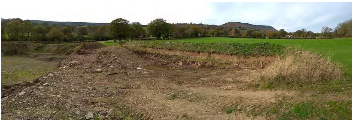
Photograph W56_1: View of site
