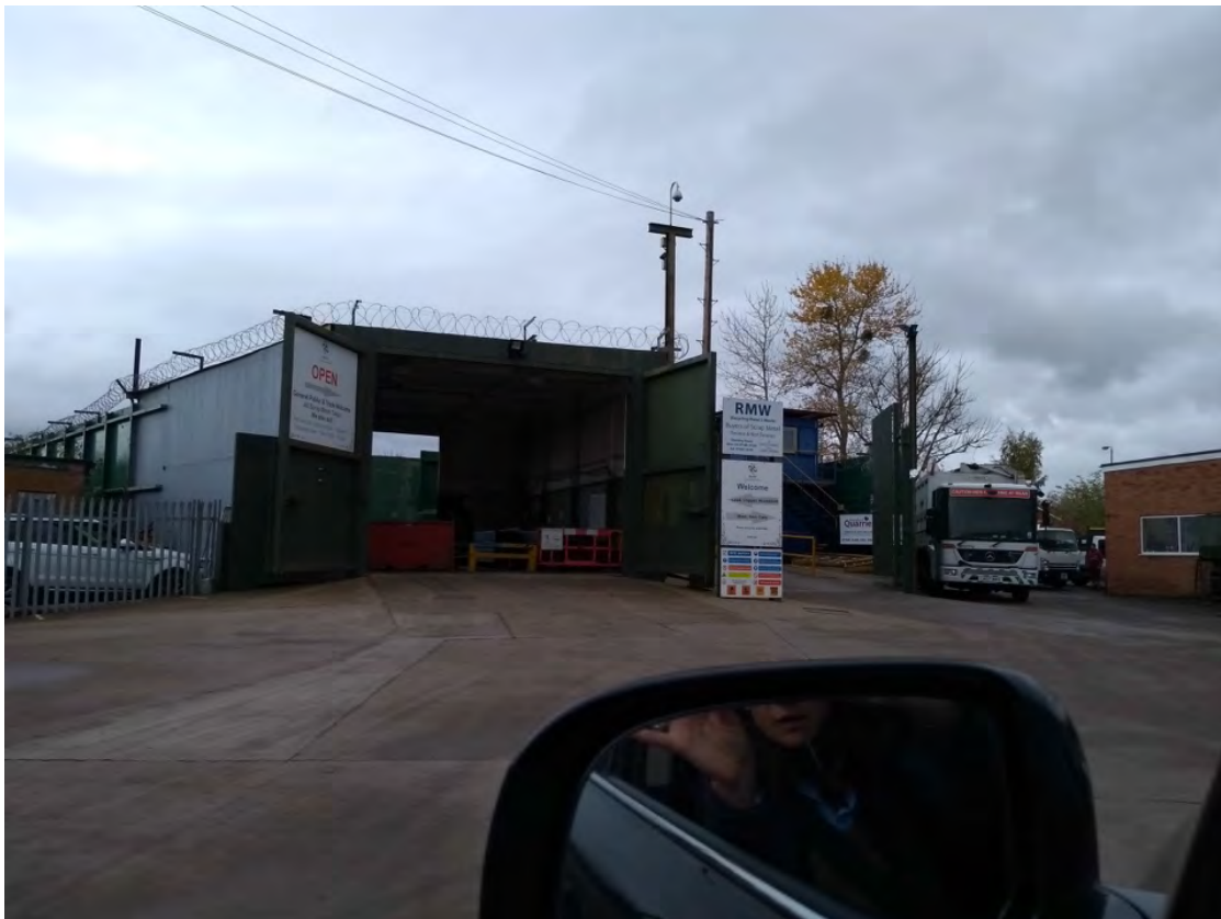
Photograph W23_1: Site entrance
