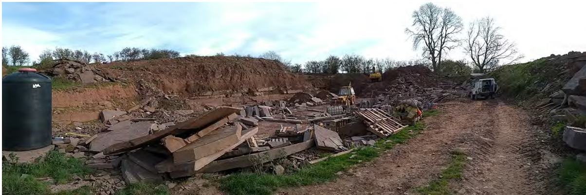
Photograph W55_1: View of site
