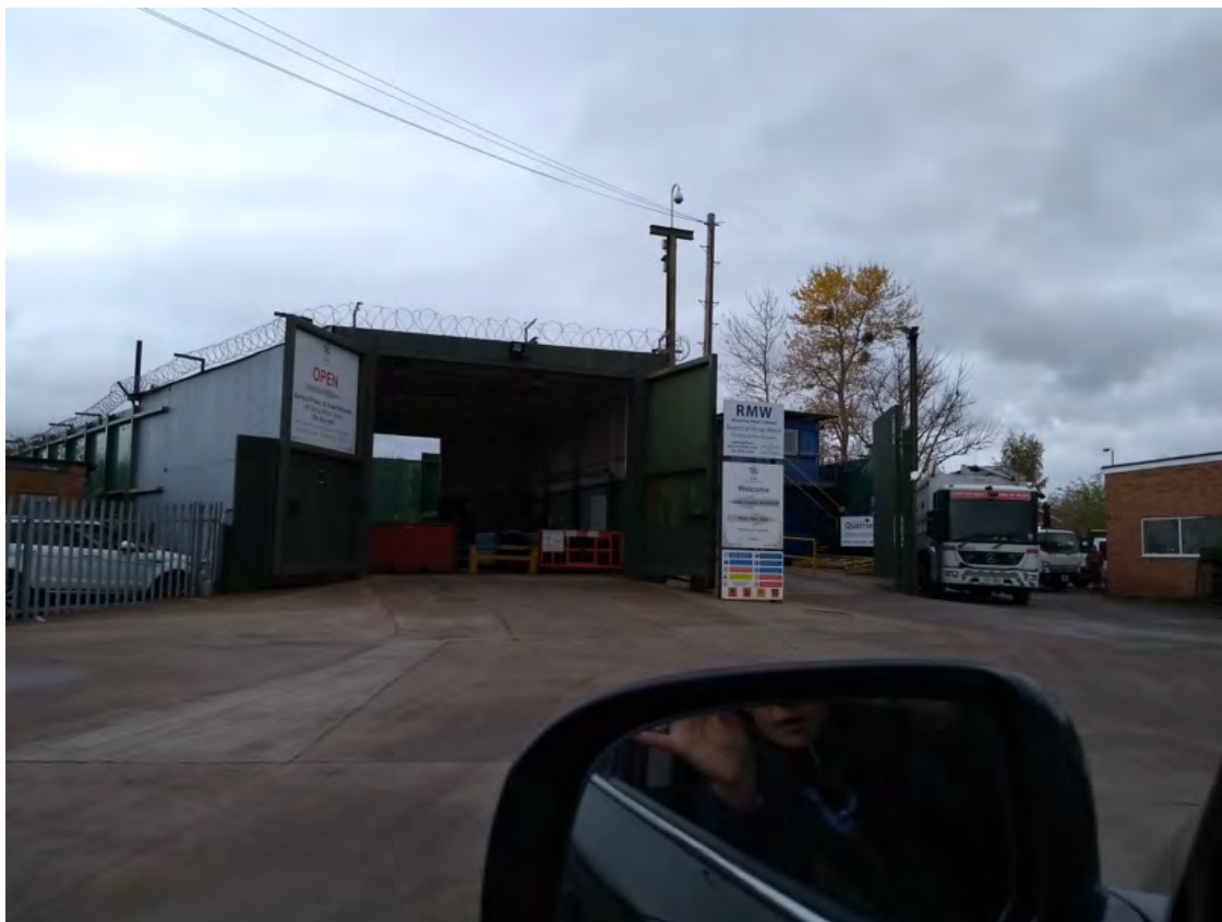
Photograph W22_1: Site entrance
