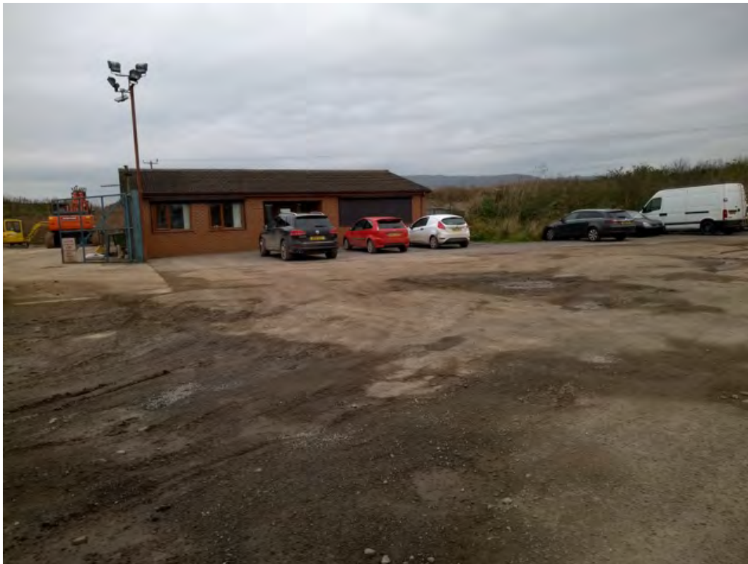
Photograph W11_1: New office on site, bunding to the right with materials processed behind.
