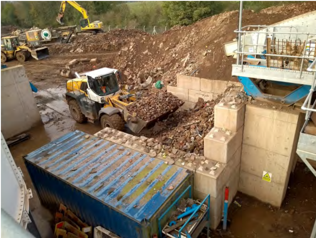
Photograph W13_2: Oversized material being taken off
