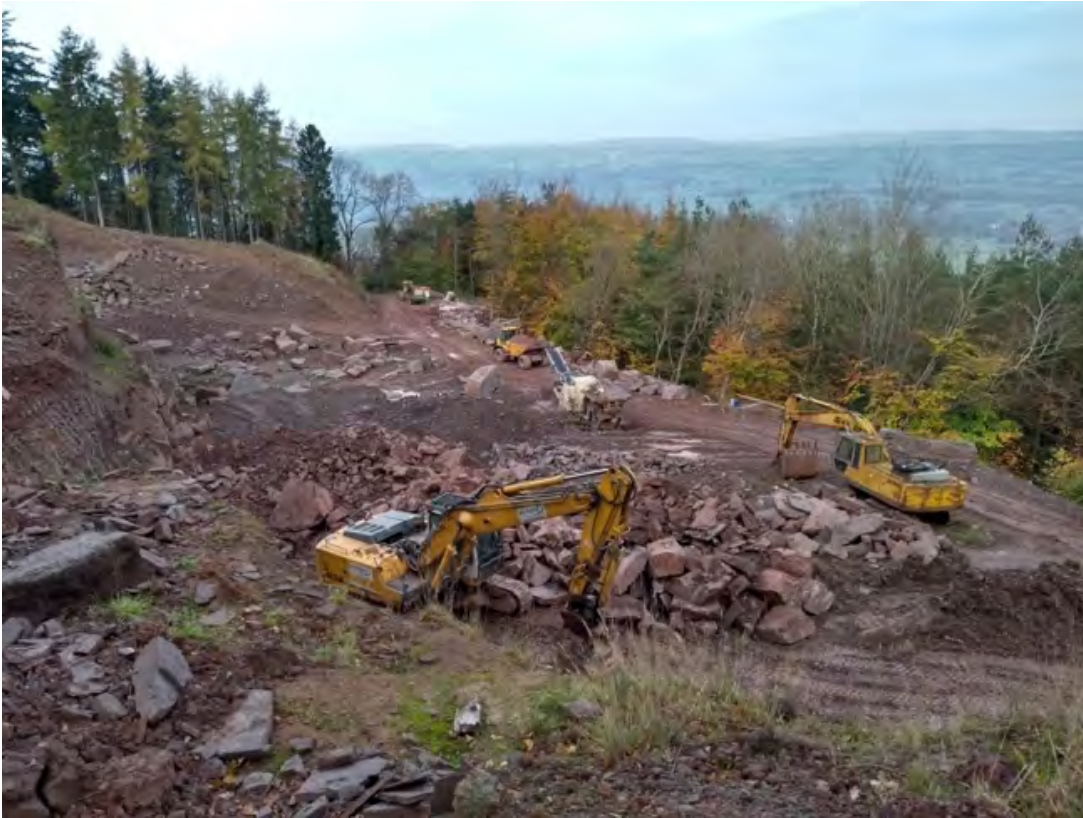
Photograph W57_1: Working face
