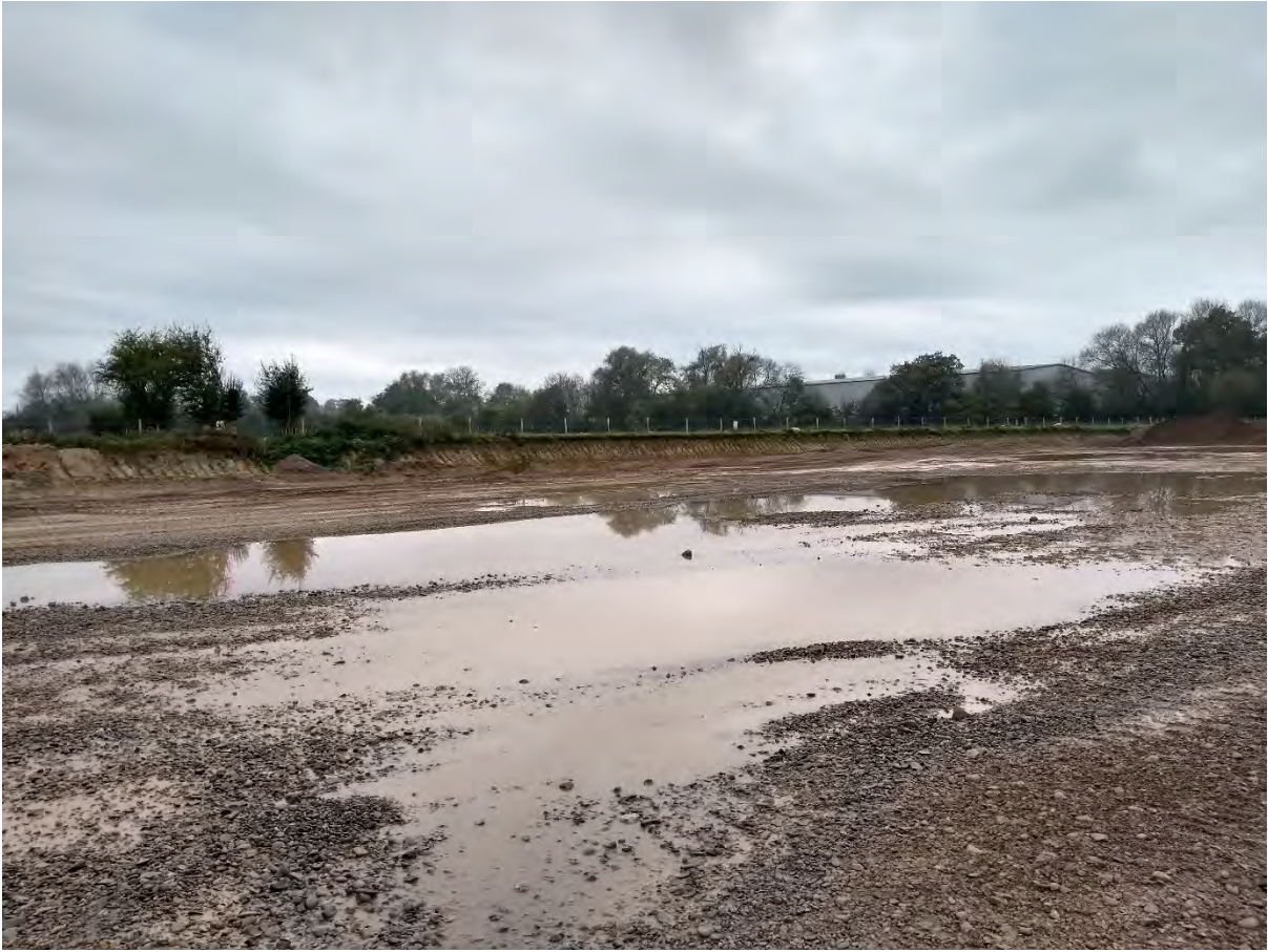
Photograph W45a_1: Working face
