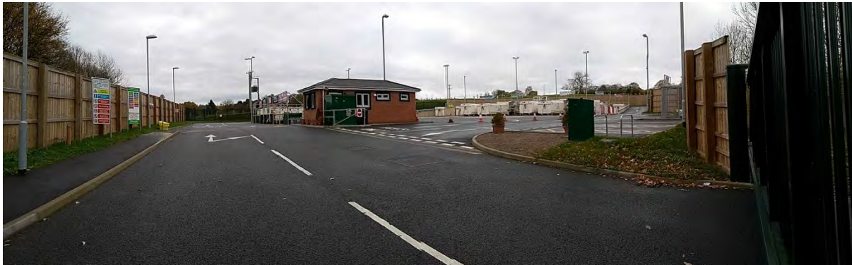
Photograph W10_1: View of site
