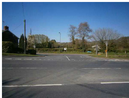
Figure 3 - A44 Bromyard Bypass and Sherford Street Junction
