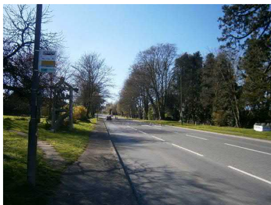
Figure 2 - A44 Bromyard Bypass (Looking Westbound)
