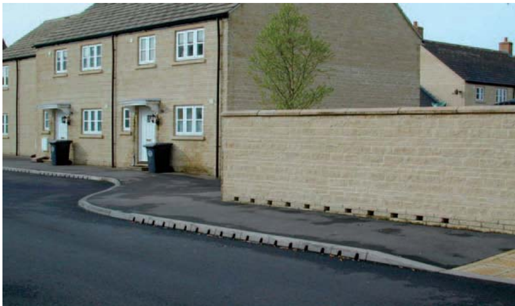
Figure 7-4 - Drainage relief openings
