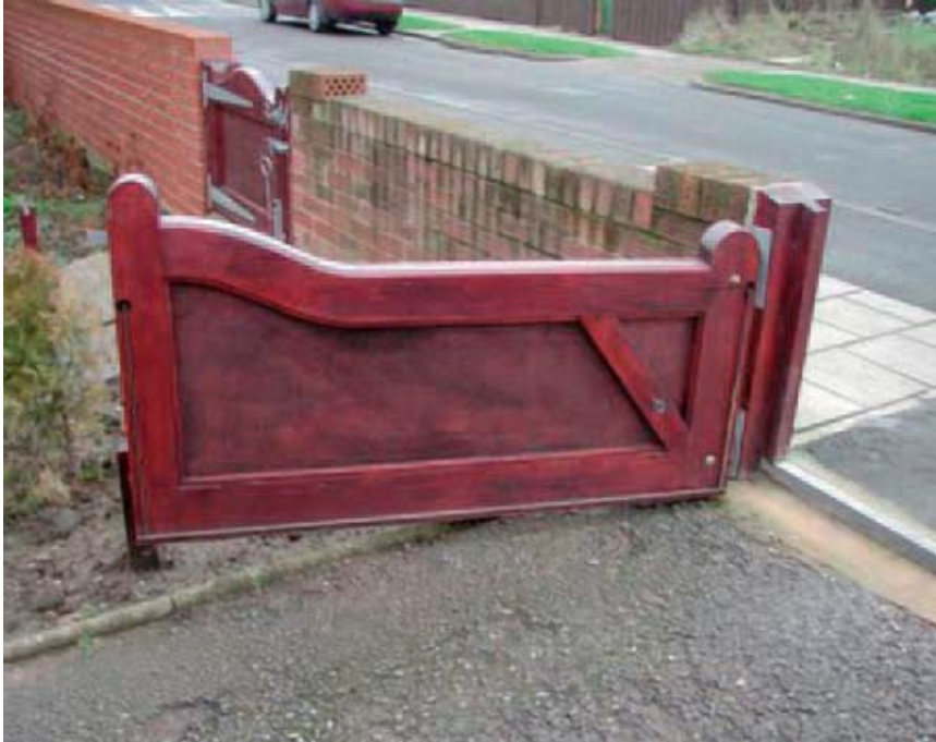
Figure 7-7 – Watertight entrance gate
