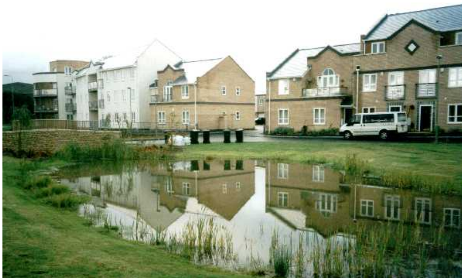
Figure 7-2 – Localised attenuation pond for new development
