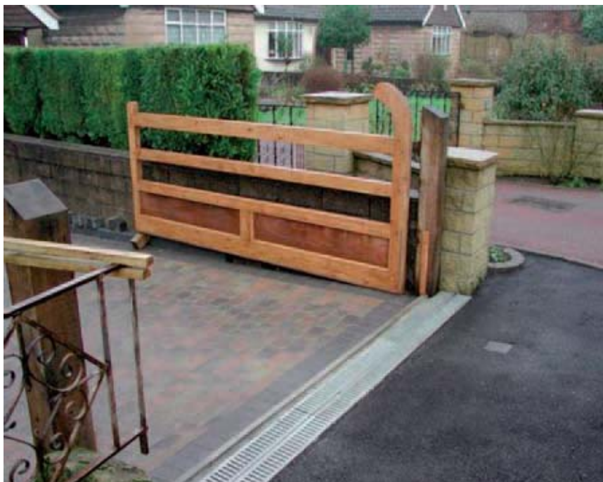
Figure 7-6 - Property boundary wall with lower sealed gate
