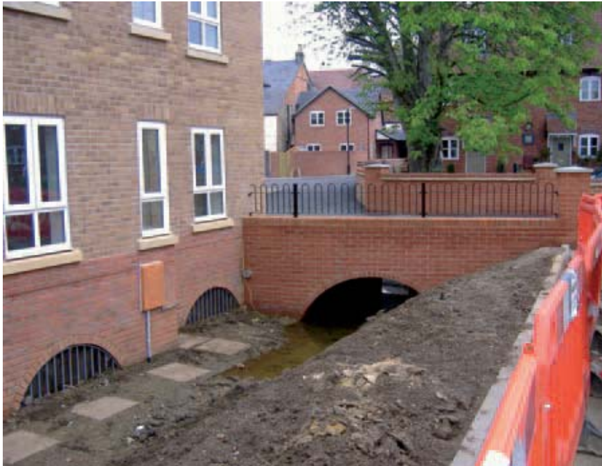
Figure 7-5 - Building Flood Management System
