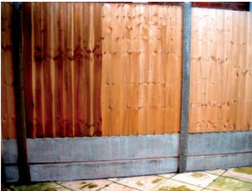
Figure 7-8 - Protected fence base with impermeable material
