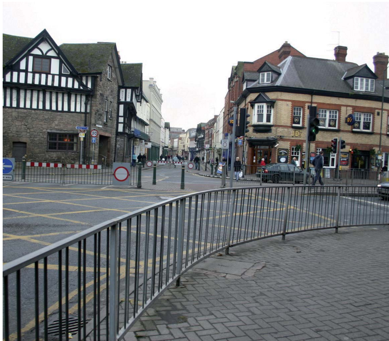
Existing guardrails in Hereford limiting movement
