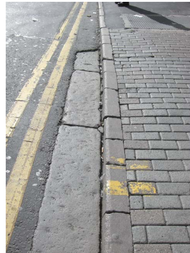
Evidence of original wide stone kerb stones
