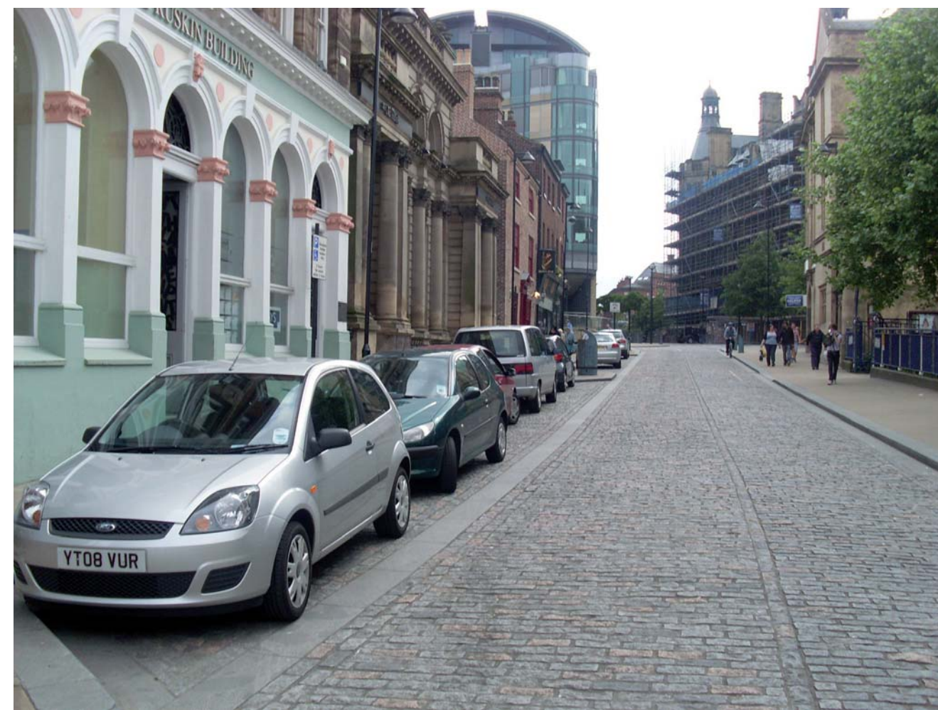
In Sheffield, careful use of materials to denote parking bays and carriageways helps to imply a slower speed is required without the use of any signage
