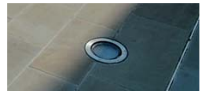
Inset lighting can highlight features such as steps, trees, public art and needs to be considered as part of the broader lighting strategy
