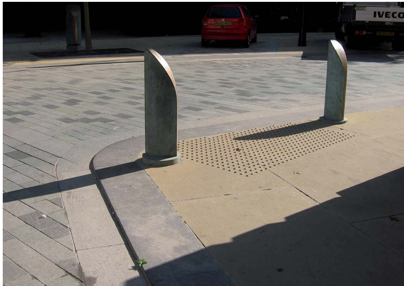
Excellent quality kerb detailing and tactile surfaces, Sheffield
