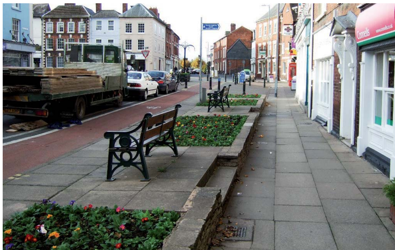
Pre-cast concrete flags on King Street in need of replacement and more recent smaller unit paviors
