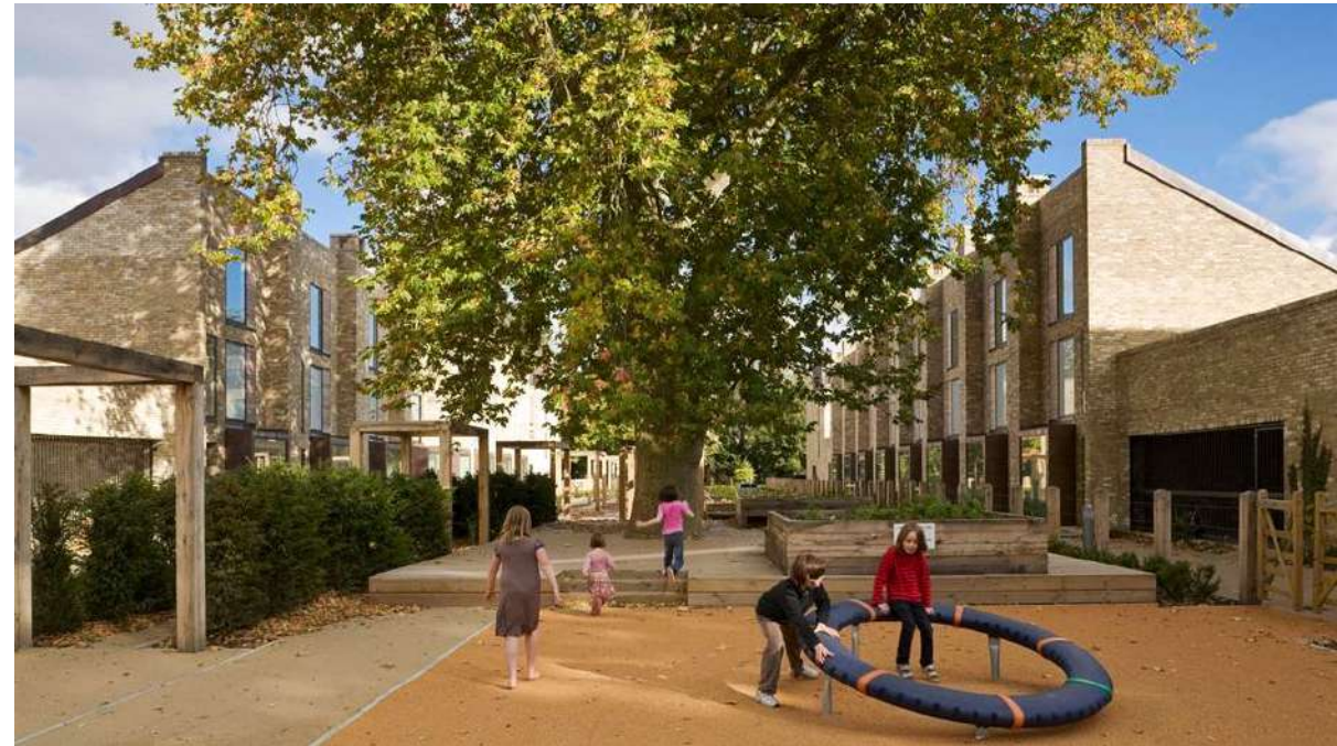
Accodia, Fielden Clegg Bradley Studios architects.
