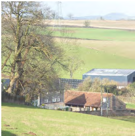
Listed converted barns, Llangrove
