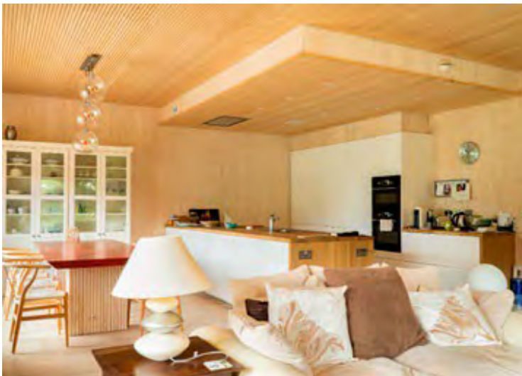
▲ Image 107: Exposed CLT Interior, Passivhaus Trust
