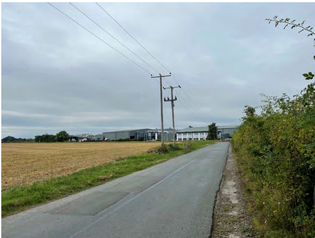
FIGURE 15: THE TORVALE INDUSTRIAL ESTATE BLOCKS ANY INTER-VISIBILITY BETWEEN THE SITE AND THE BARROW CEMETERY TO THE WEST
