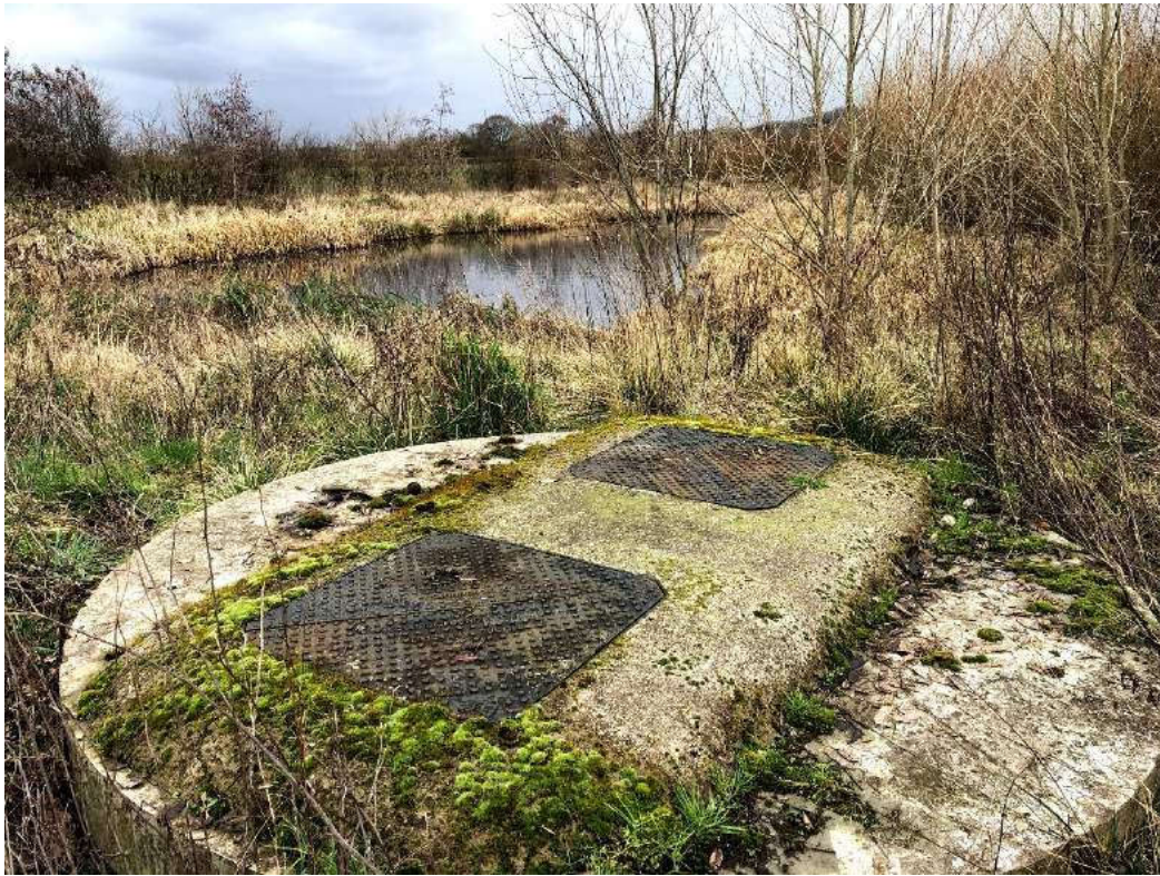
Figure 4-4 Flow control from the final attenuation pond to the wetland
