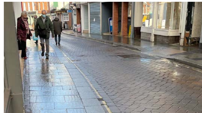
Narrow pavements and high kerbs
