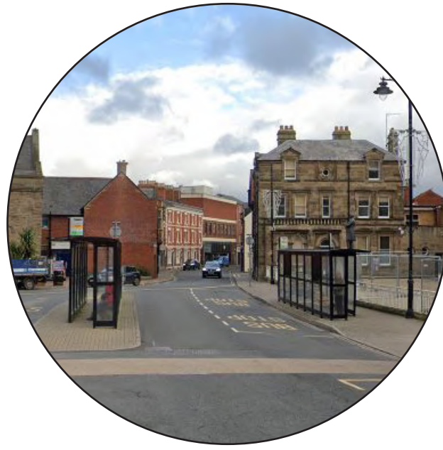
Existing bus shelters outside Shire Hall
