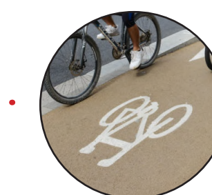
Buff surface treatment on dedicated cycle path.
