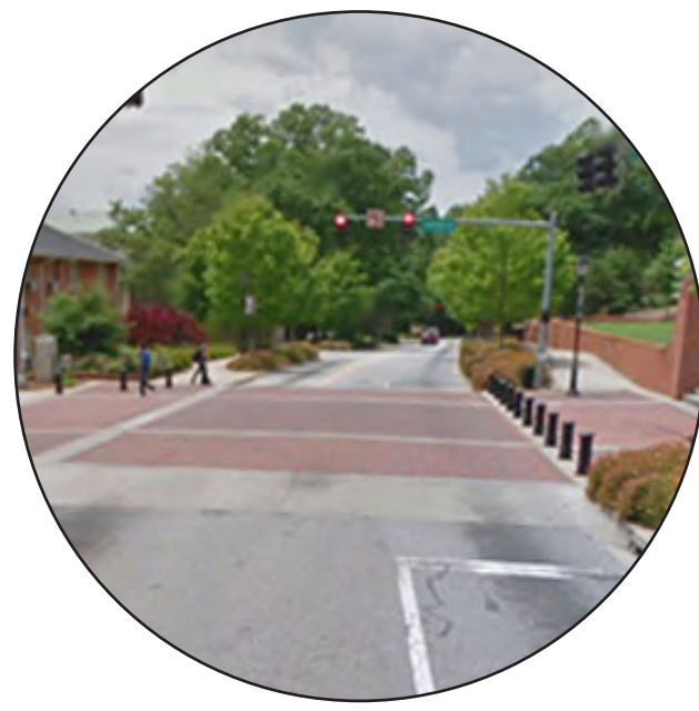
Raised table at junction with imprint detail
