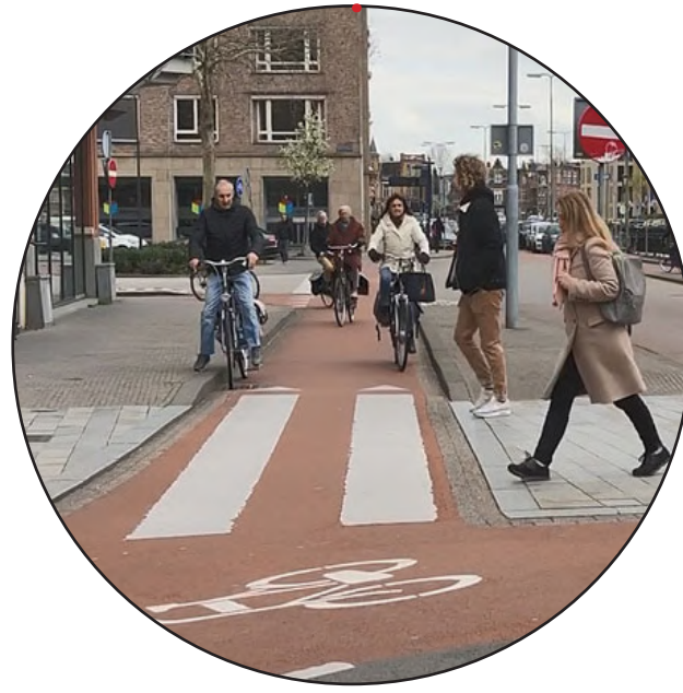
Pedestrian crossing over cycle lane
